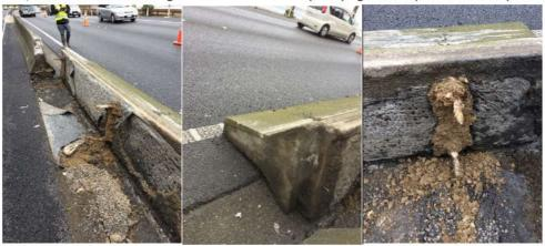
In both examples the New Jersey Barrier units were not connected to the adjacent units and ground pins were in poor condition, rusted and only embedded in the in-situ ground. This resulted in there being no ribbon strength along the length of the new jersey barrier or ability of the individual units to resist the impact loads.
