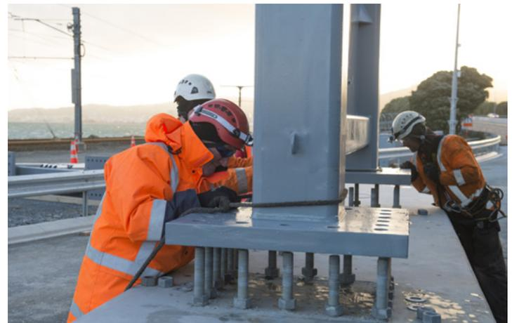
Lining up the 36 bolts while lowering the 6 tonne gantry leg into place.
