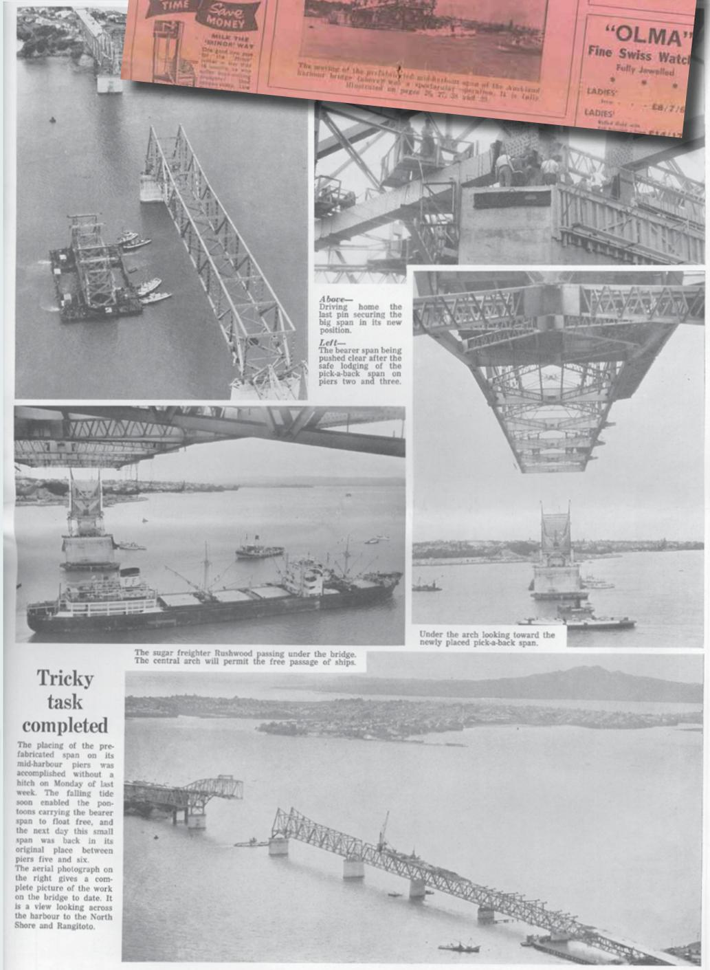
Above— Driving home the last pin securing the big span in its new position.
