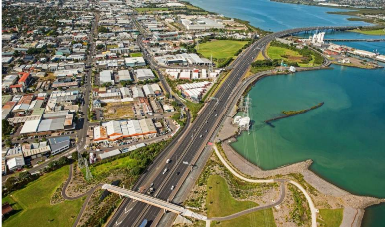
Figure 11-5: Looking south on SH20 with Māngere Inlet in the distance (present day)
