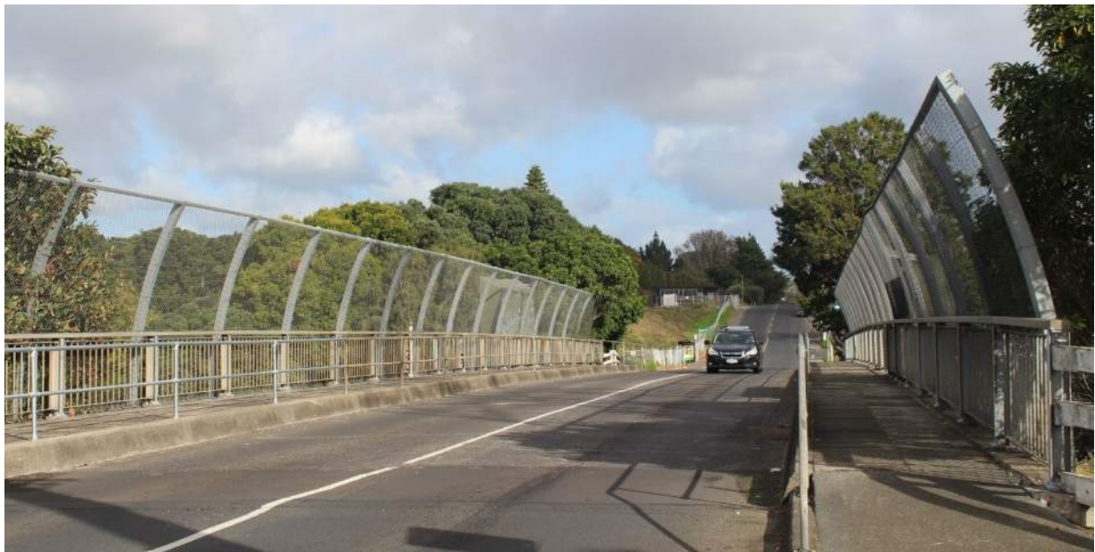
Figure 11-6: Panama Road Bridge (present day)
