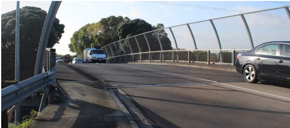
Figure 11-7: Princes Street overbridge (present day)
