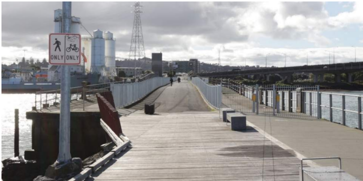
Figure 11-8: View of Old Māngere Bridge looking north towards Onehunga
