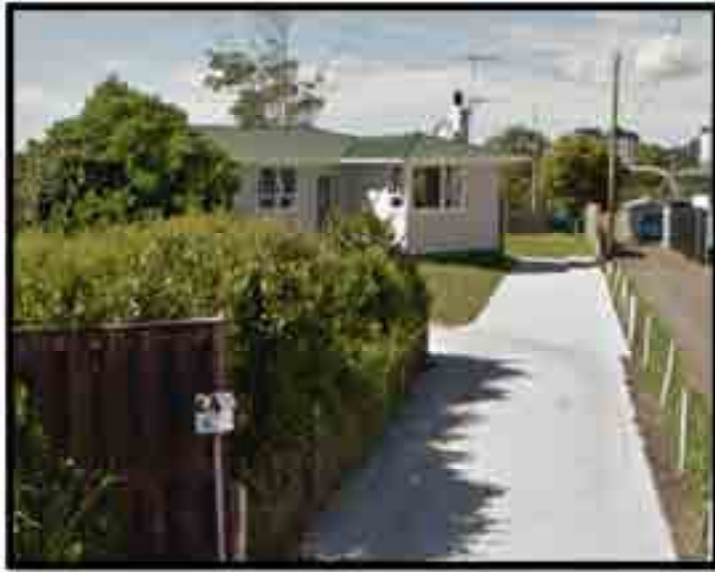
Figure 30: 16 Coppins Road. Street view.
