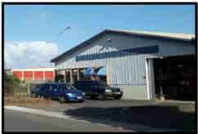
Figure 3: 2 to 2a Hill Street. Hill Street frontage.
