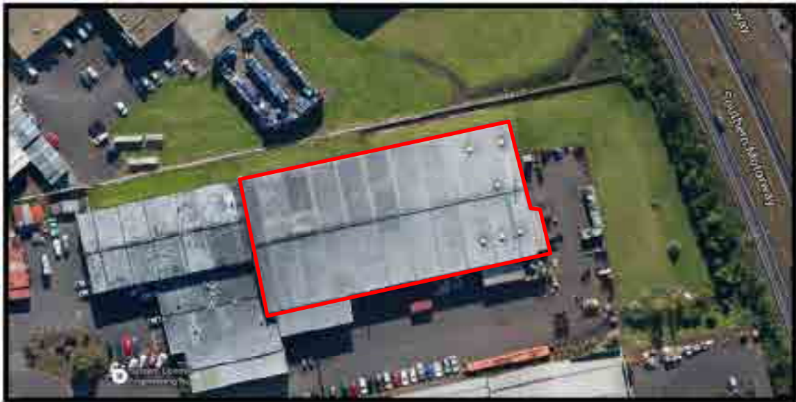
Figure 19: 7 Carmont Place. Satellite view.
