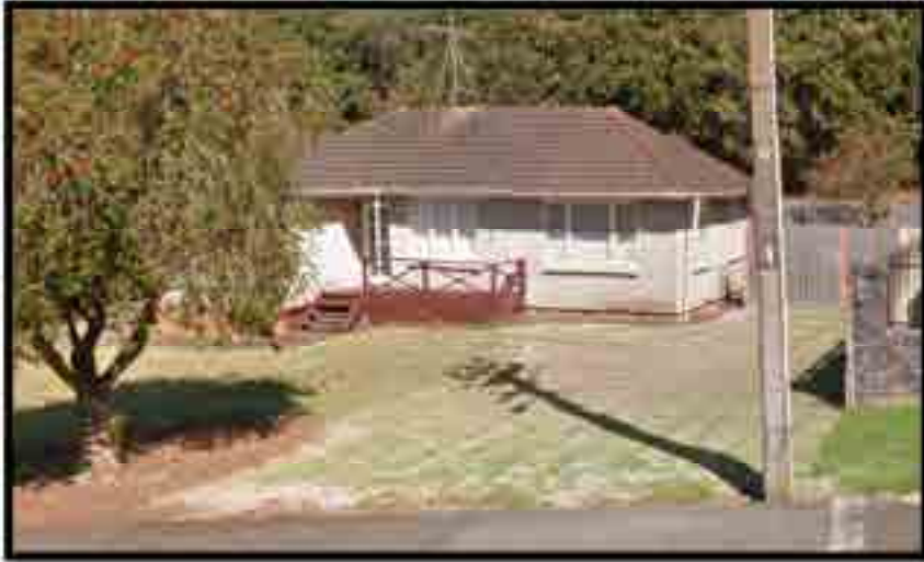
Figure 28: 110 Hillside Road. Street view.
