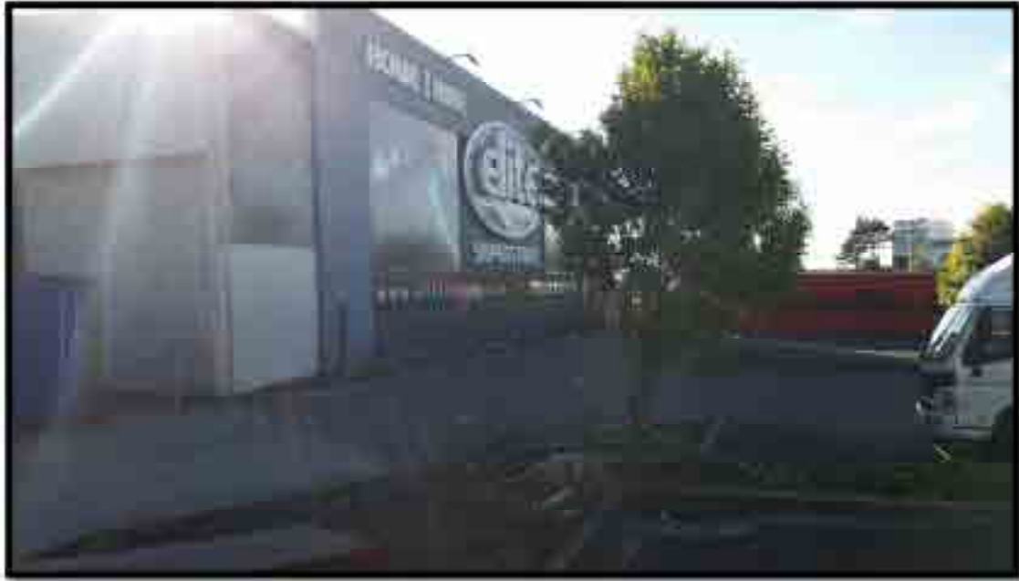
Figure 22: 11 George Bourke Drive. View from car park.
