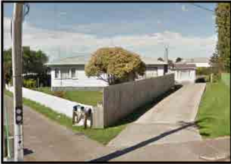
Figure 32: 14 Coppins Road. Street view.
