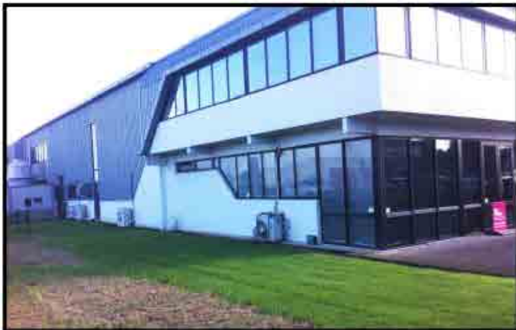
Figure 5: 3-5 Gloucester Park Road. . Neilson Street frontage.
