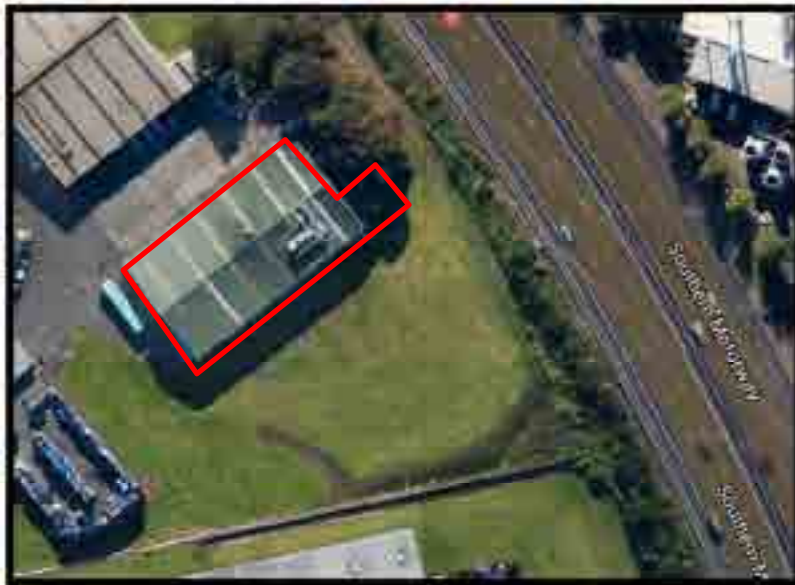
Figure 17: 5 Monahan Road (PPG Industries). Satellite view.
