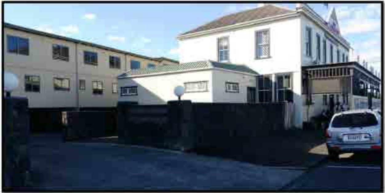
Specific Building B-ID 4: 40 Victoria Street, Onehunga
