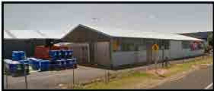
Figure 2: 2 to 2a Hill Street. Neilson Street frontage.
