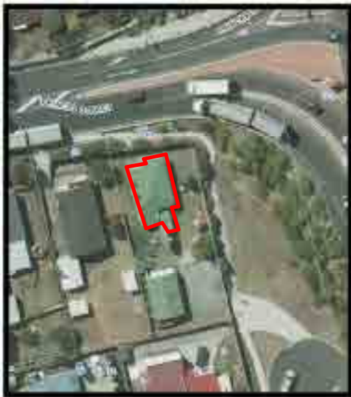
Figure 37: 95 Princes Street. Satellite view.
