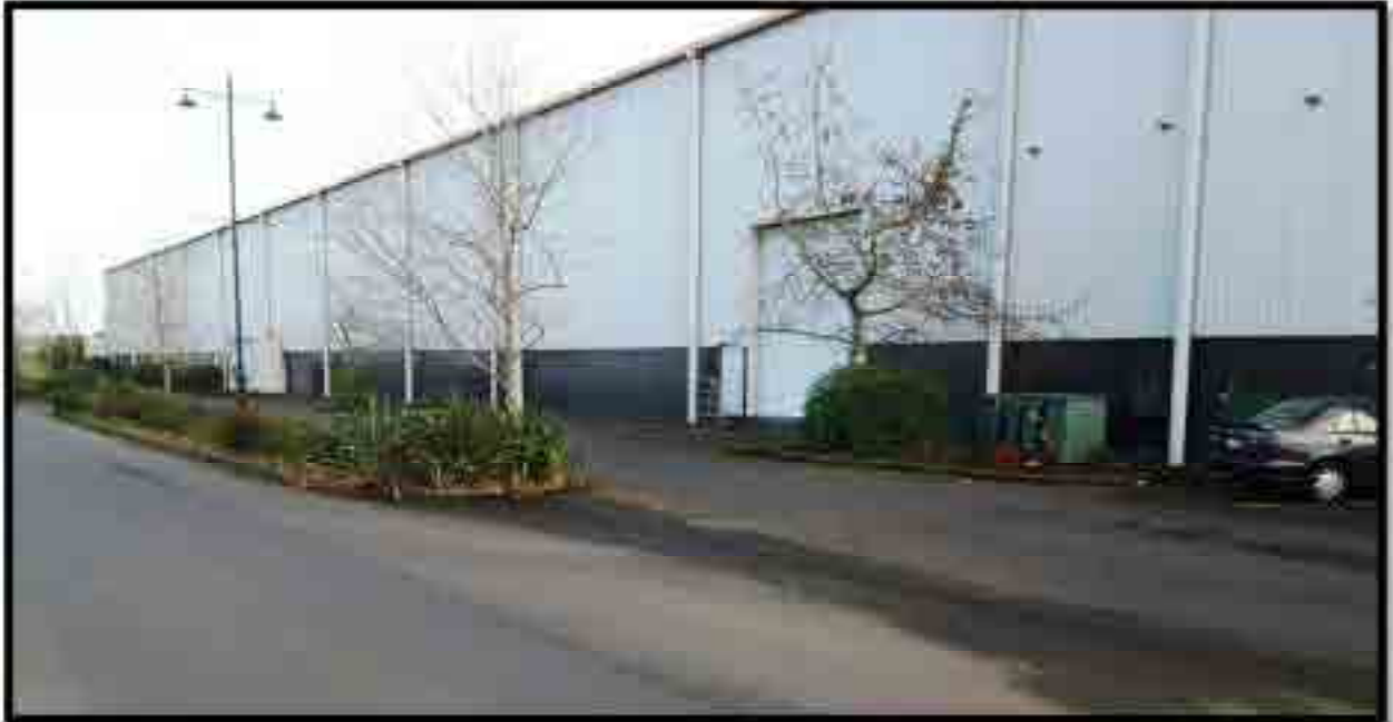
Figure 12: 69 Captain Springs Road. Street view.
