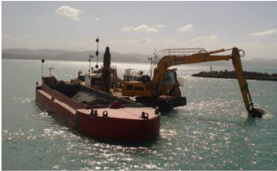
Figure F2: Mechanical (backhoe) Dredger loading a Receiving Barge
