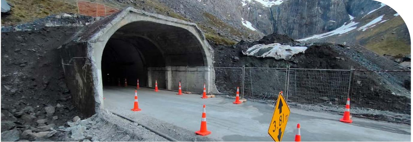
A steady stream of the approximately 150 pre-cast concrete modules required for the new shelter are regularly arriving on site. The wall on the southern side of the shelter is clearly visible as you can see in the photo below. These modules are made off-site then transported to the tunnel for assembly.
