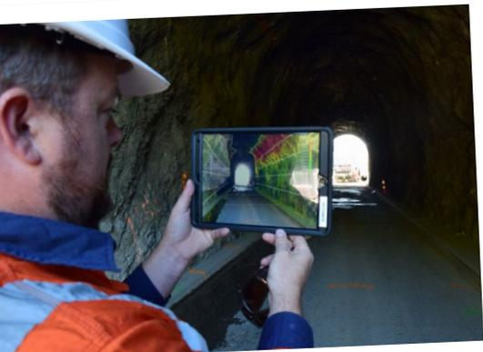
Pictured is Chris Souter, viewing the app in the Raramai South tunnel. The colours represent the amount of material, which needs to be removed from the existing tunnel surface to reach the desired 'new' designed dimensions (ranging from no colour, which is already wide enough, through a range all the way to red - which is more than a metre to remove).
