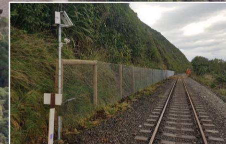
We're protecting the rail network by installing rockfall protection to stop rock or other material falling onto the tracks. We have installed in some areas detection fences, which automatically let train control know if any material has fallen on the track so we can respond as quickly as possible.
