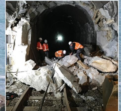
Twenty rail tunnels along the route needed repairing from earthquake damage. We have repaired 15 of these and are continuing to work on the final five.
