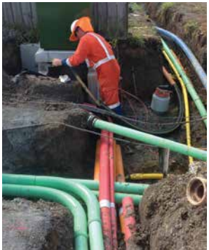
This photo: Pavement construction Left: Utilities being relocated underground
