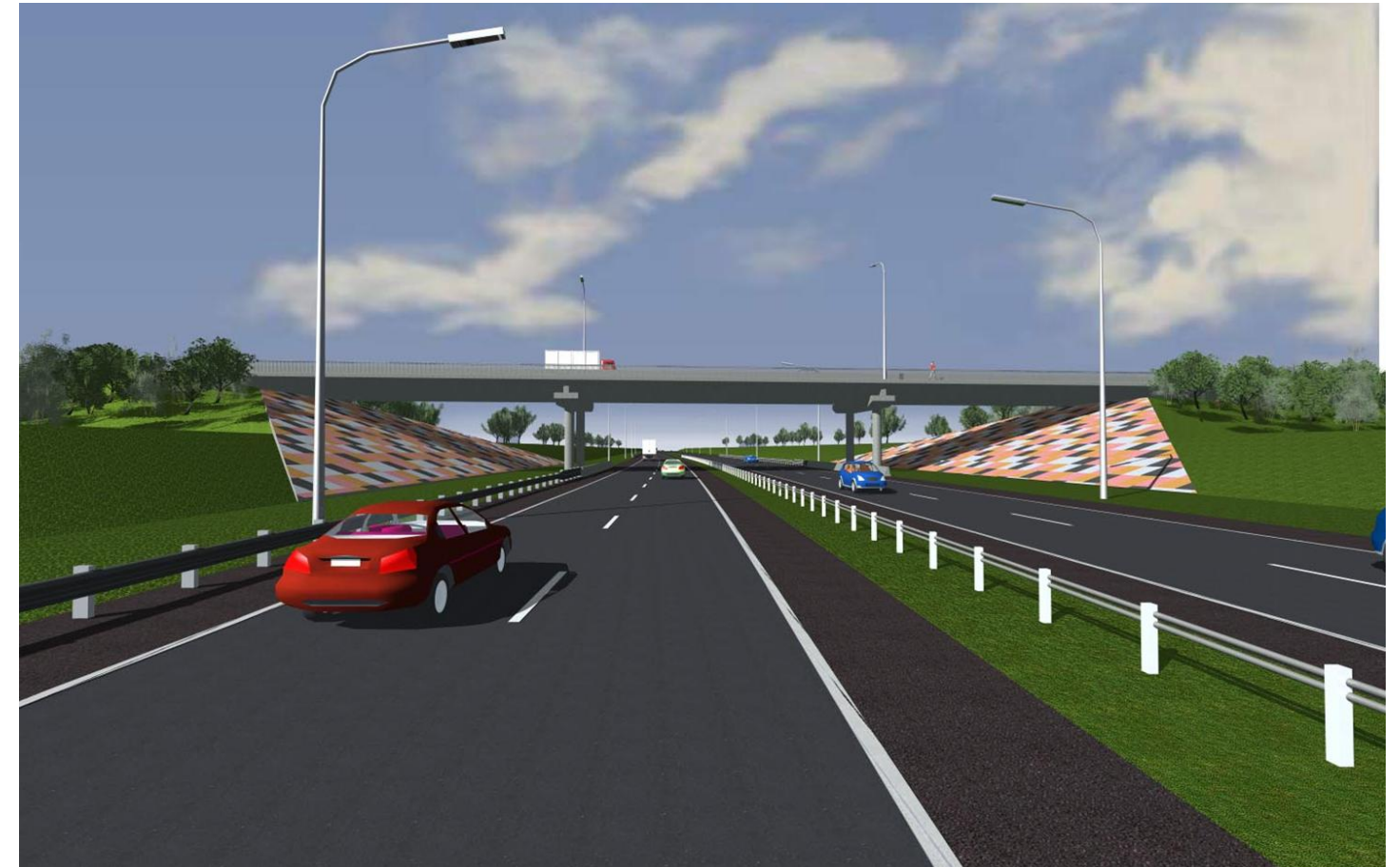
Figure 12b: View from CSM2 southbound carriage way showing super tee structure, open spill through and abutment slope treatment.
