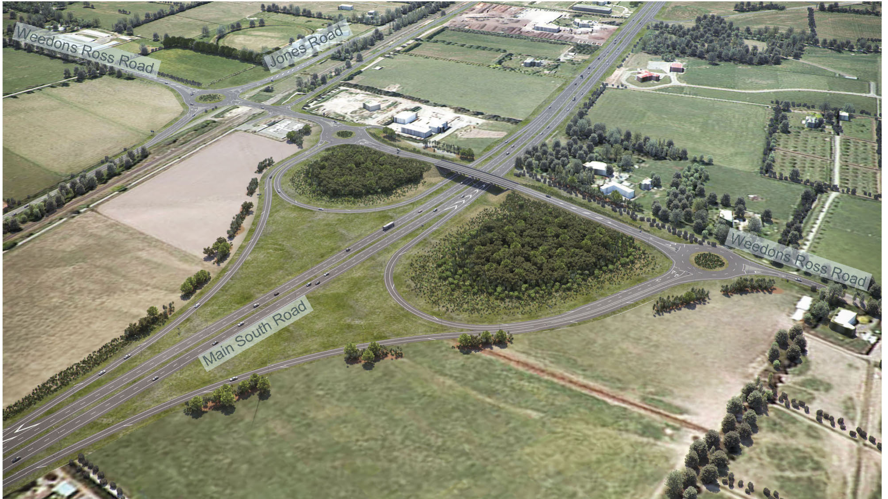
Figure 29: Weedons Road Interchange
