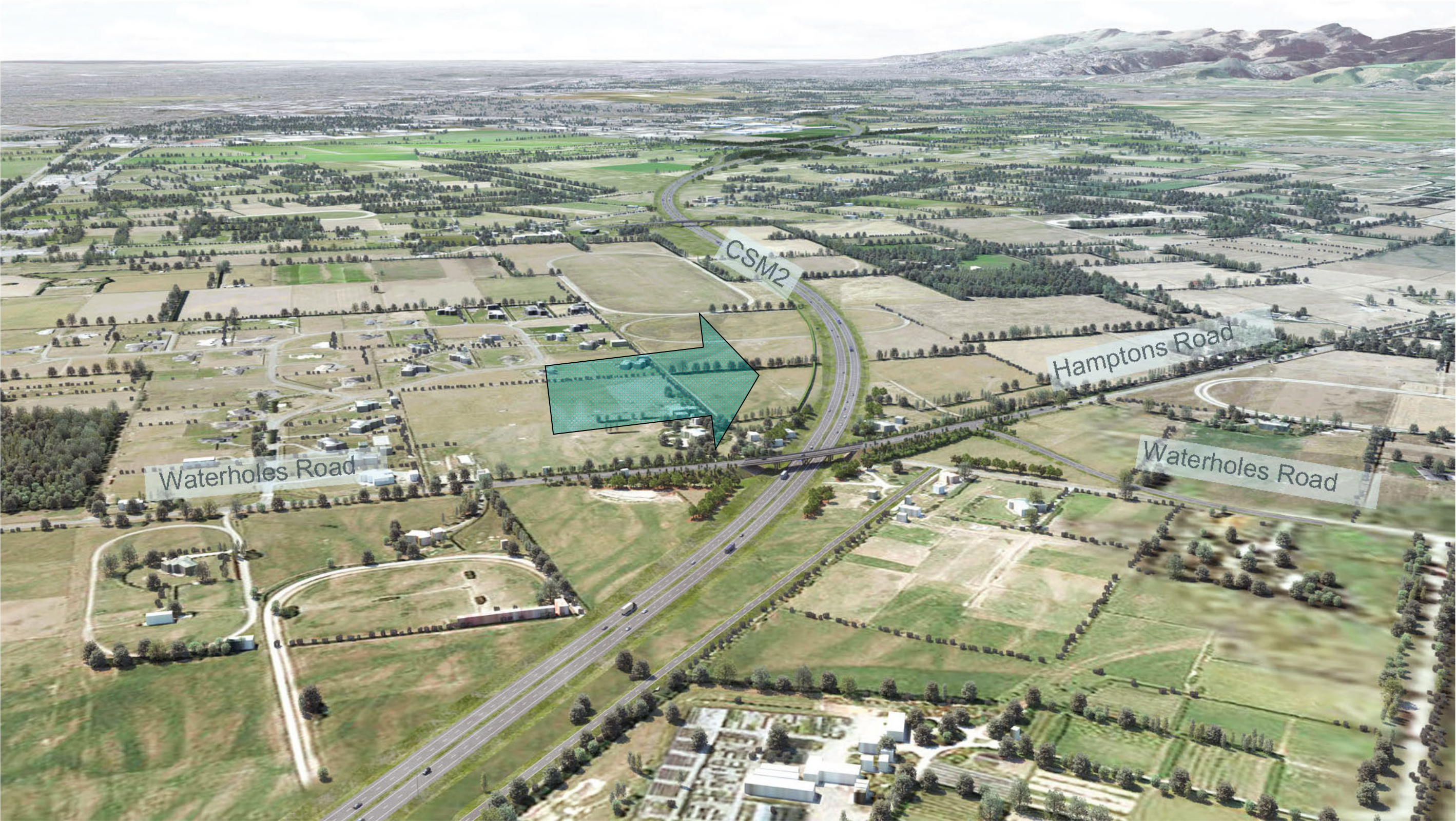
Figure 25: Waterholes Road Overbridge (looking north)
