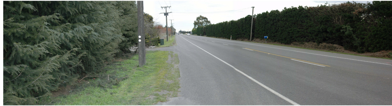
Viewpoint 9: Looking southwest along SH1 approximately 350 metres from the Robinsons Road overpass of the MSRFL proposal.
