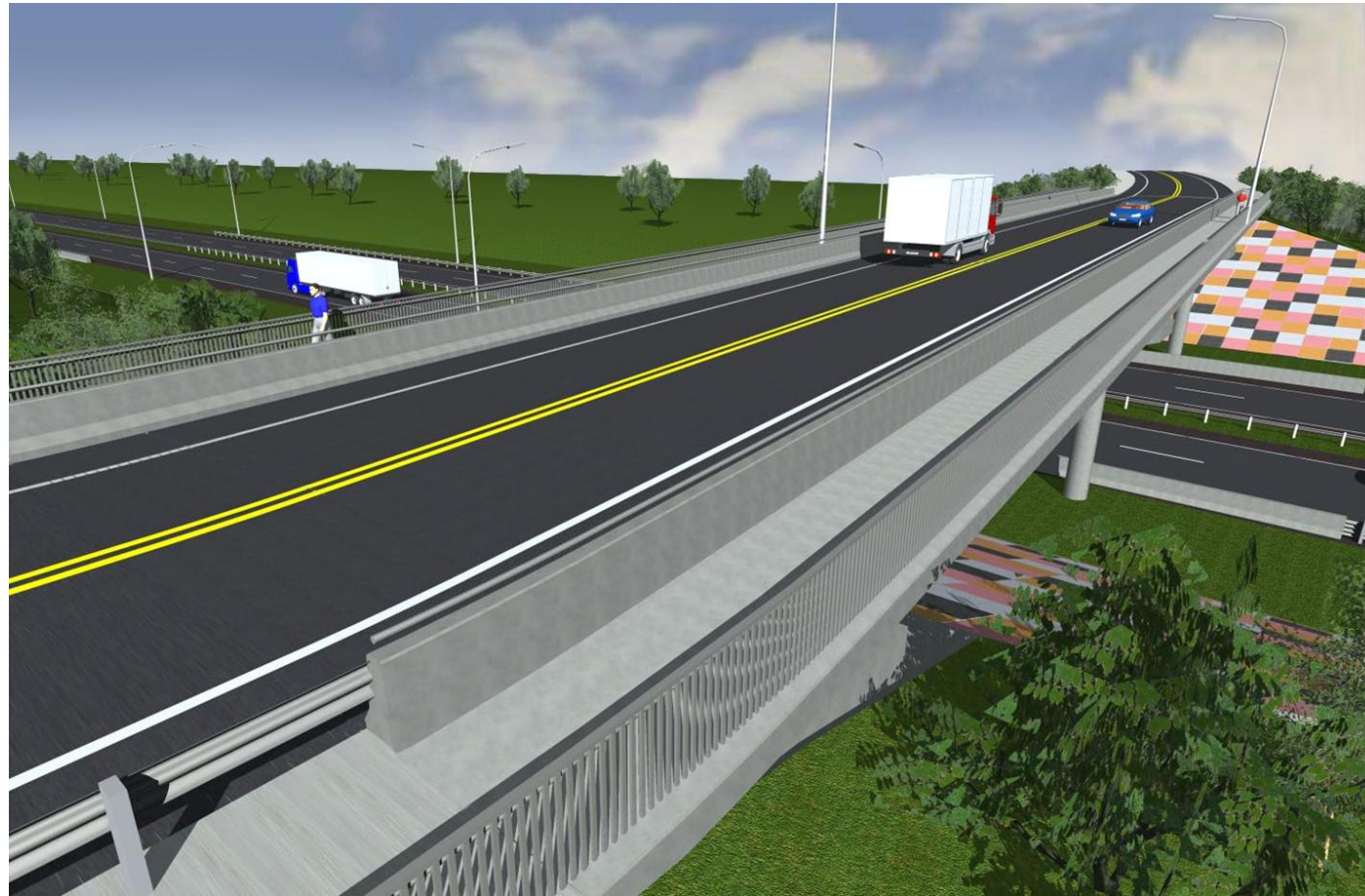
Figure 12a: Artist's impression of Trents Road Bridge showing open steel balustrade to footpath edge and concrete safety barrier between footpath and local road.
