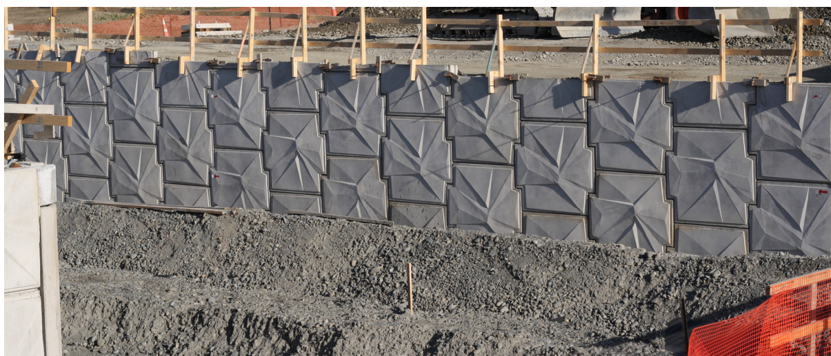
Figure 13: Design images of Barrington Street Overpass (local road under) from CSM1 showing precast MSE panels with textured finish and photograph of MSE panels under construction. The Robinsons Road overpass matches these design features. Images courtesy Fulton Hogan and Jasmx (left)
