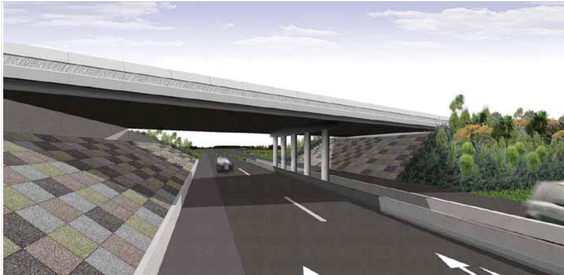
Figure 10: Artist's impression of Curletts Road Bridge in CSM1 showing abutment slope finish. Image courtesy Fulton Hogan and Jasmax
