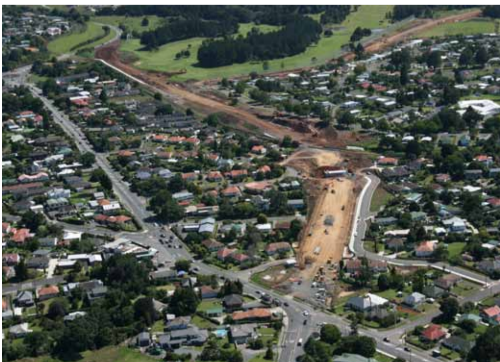
Under construction, January 2011
