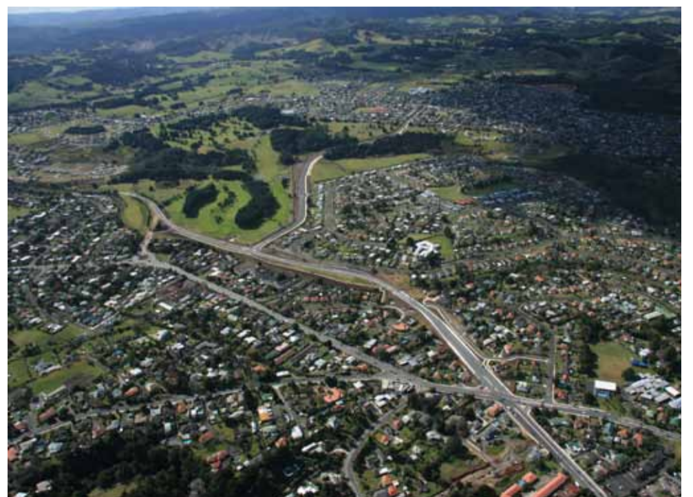
Under construction, August 2011
