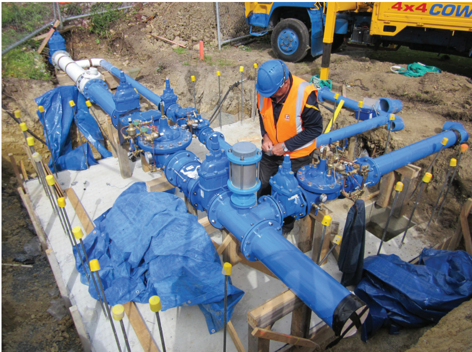
New water chamber being constructed on SH14, behind the new footpath
