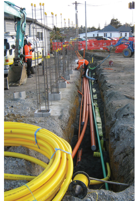
Laying new underground services
