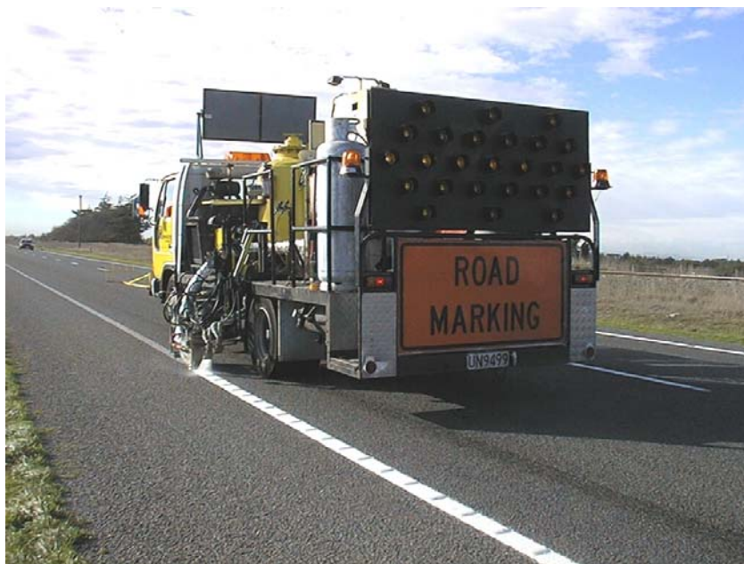
Figure 4.1 Thermoplastic being laid on State Highway 1, south of Christchurch in 2001.
