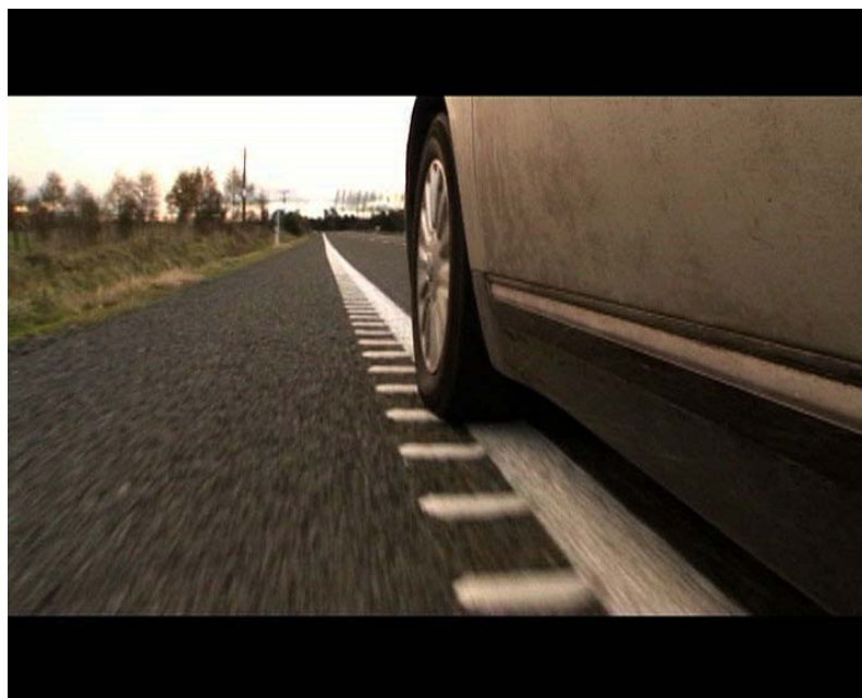
Figure 5.1 ATP cold applied plastic bumps adjacent to a continuous line (Source: Rob Dunne, Damar Industries Ltd).
