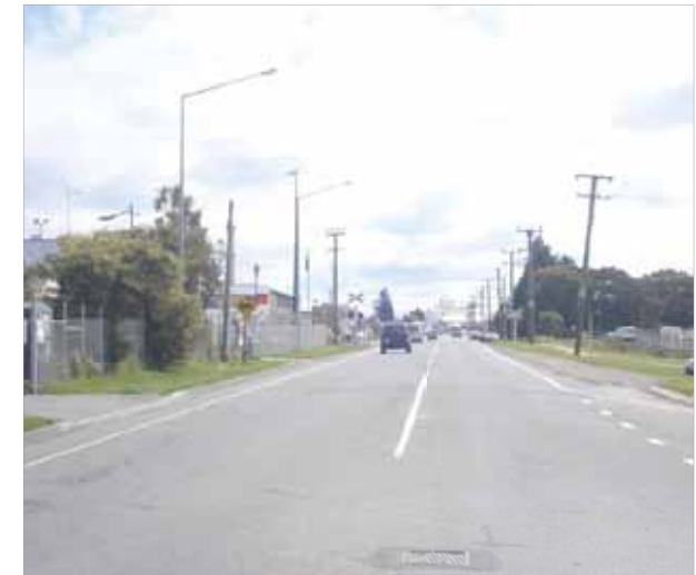
Figure 19: Lack of vegetation on Halswell Junction Road
