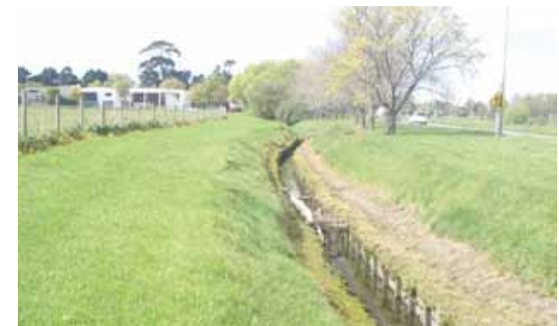
Figure 15: Existing conditions at Curletts Drain
