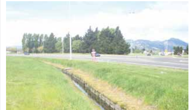
Figure 9: View of the Port Hills at Curletts Road
