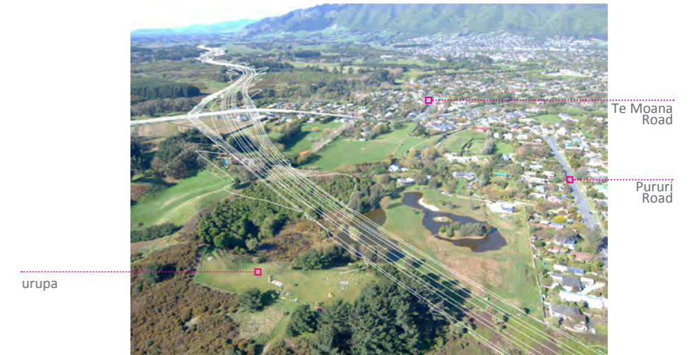
Figure 81 Waikanae option (preferred) which show the Expressway alignment avoiding houses on Pururi Road
