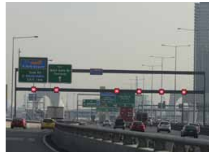
Photo 4.27: Orthogonal signage gantry
