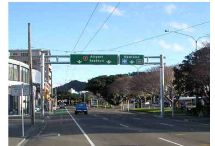
Photo 4.30: Well integrated girder and signage panels
