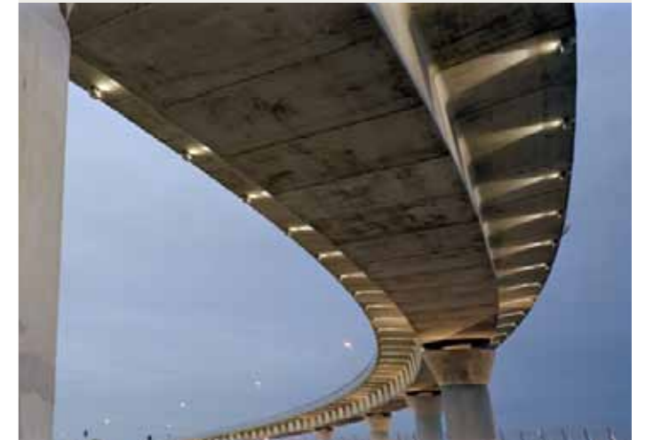
Photo 4.3: Feature lighting for gateway location
