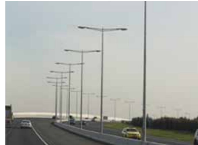
Photo 4.26: Simple orthogonal light standards
