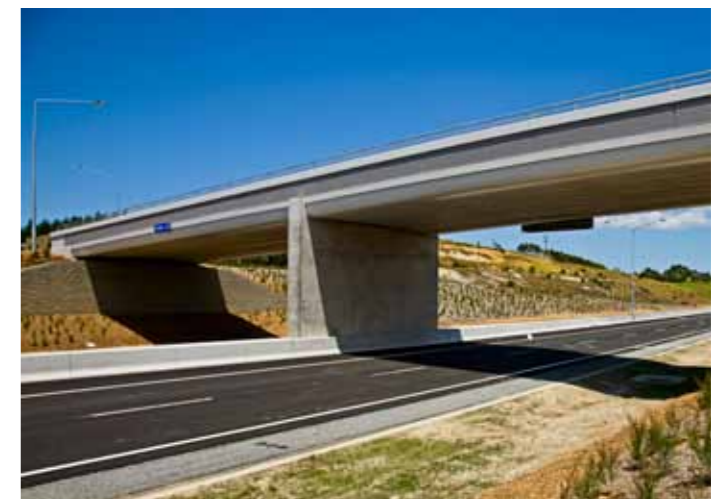
Photo 4.5: Bridge barrier extends down to conceal girder
