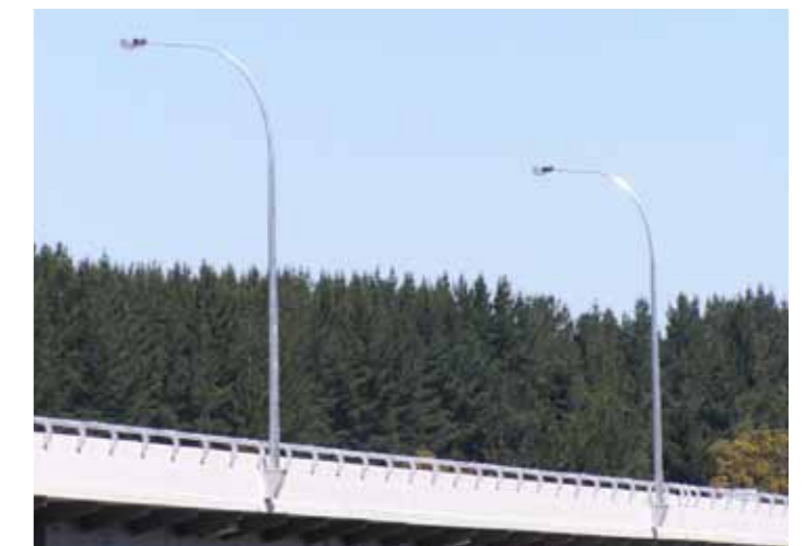
Photo 4.31: Light columns mounted to side of bridge
