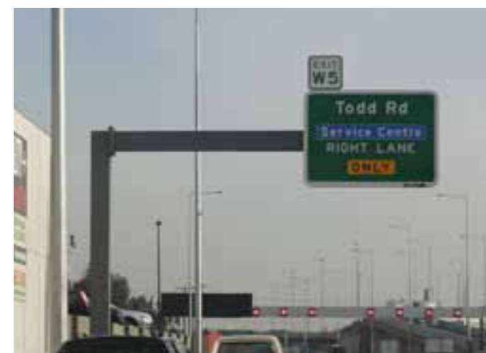
Photo 4.28: Orthogonal signage post
