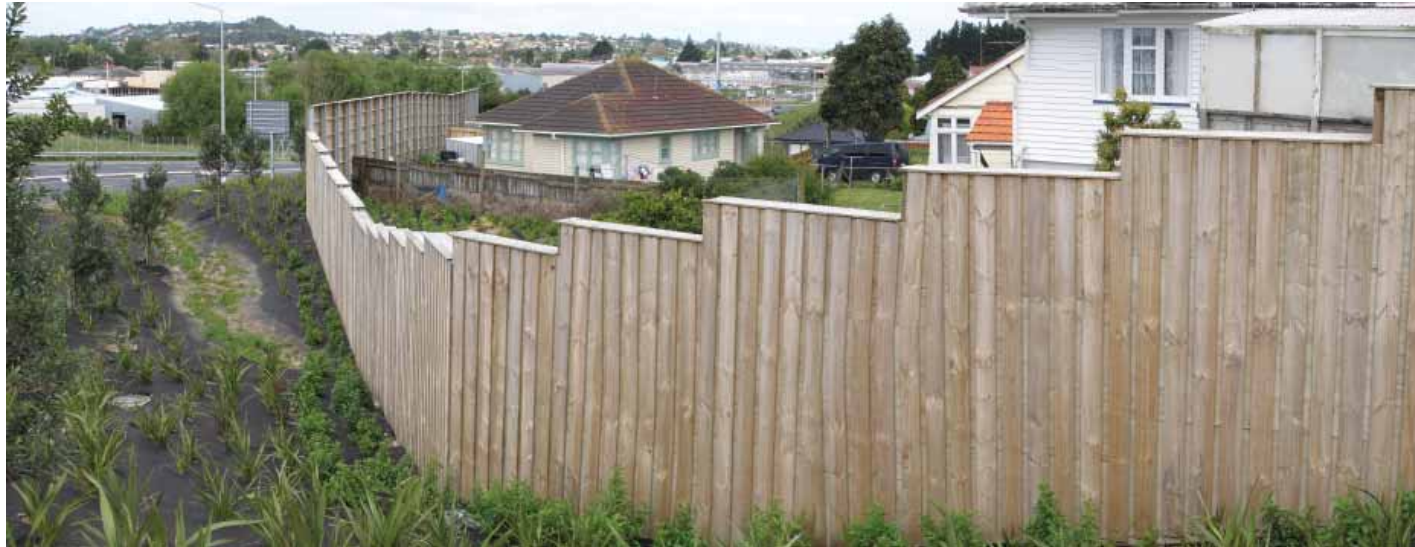
Figure C-10.76: Photo 10-5 View of existing noise walls and planting at Maioro Street extension
