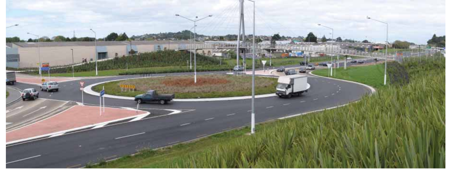
Figure C-10.78: Photo 10-7 View from Ernie Pinches Street towards temporary roundabout and pedestrian overbridge
