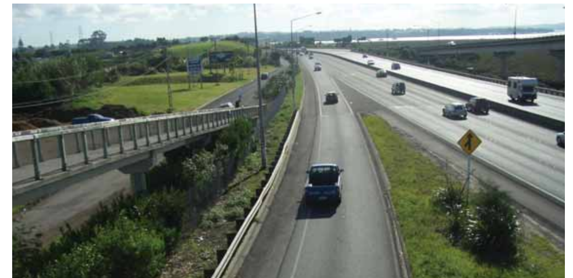
Figure C-3.3: Photo 3-2 Existing view westwards from Patiki Photo
