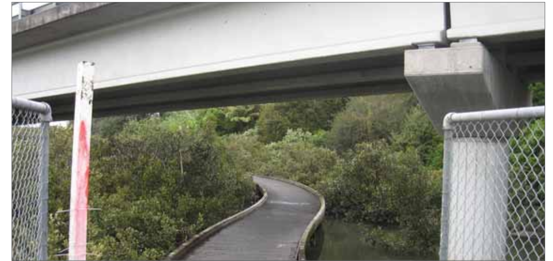
Figure C-3.9: Photo 3-4 Existing cycleway boardwalk underneath Rosebank off-ramp
