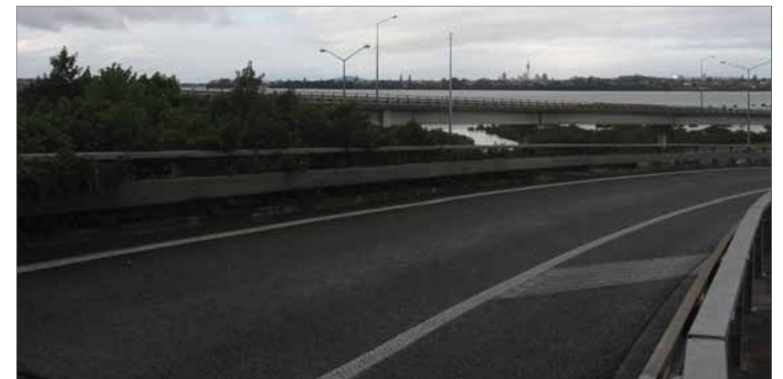
Figure C-3.11: Photo 3-6 Existing view westbound, between Rosebank ramps
