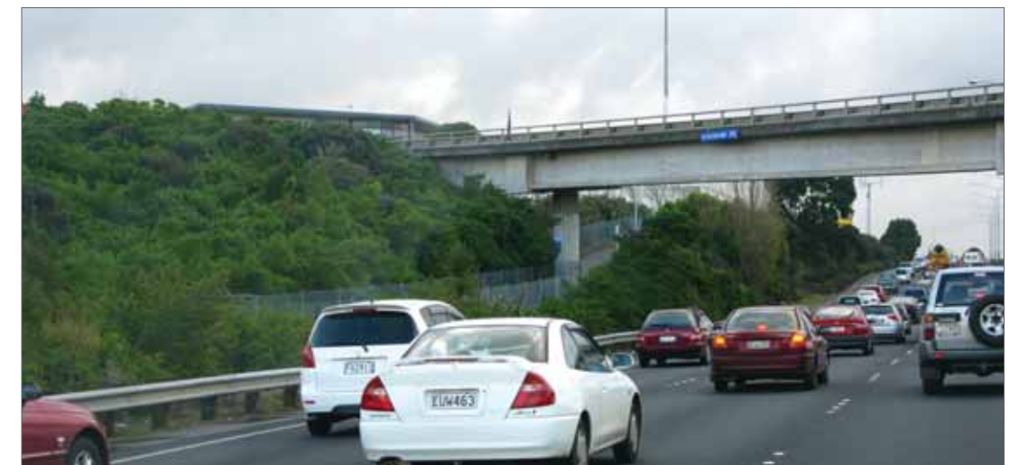
Figure C-3.10: Photo 3-5 Existing view westbound, between Rosebank ramps
