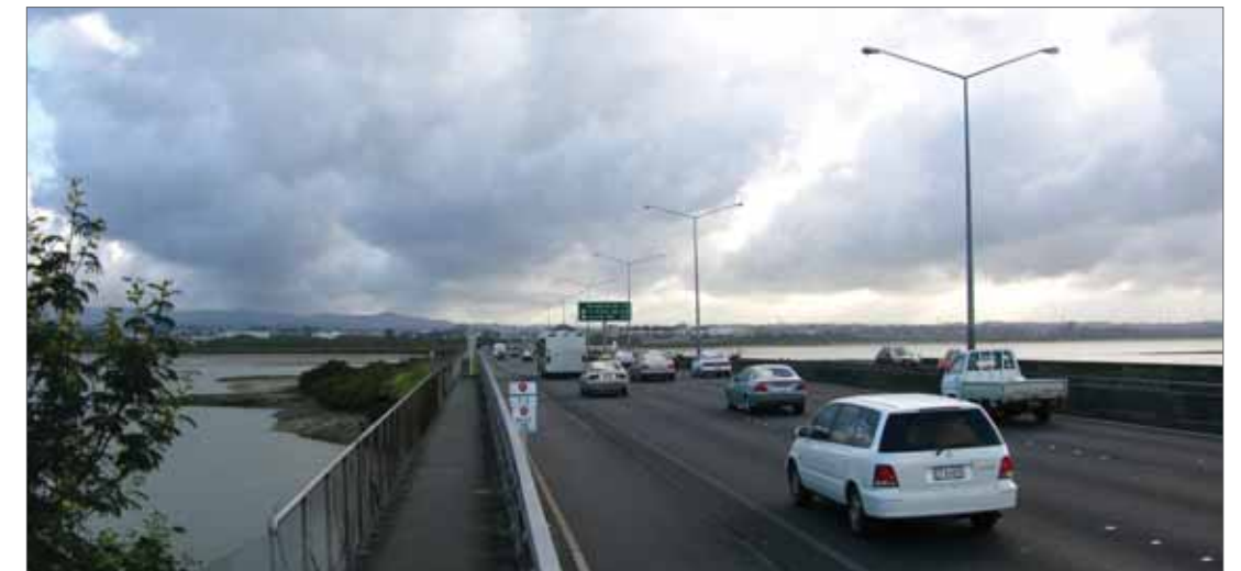
Figure C-4.15: Photo 4-7 Existing view west on Rosebank bridge
