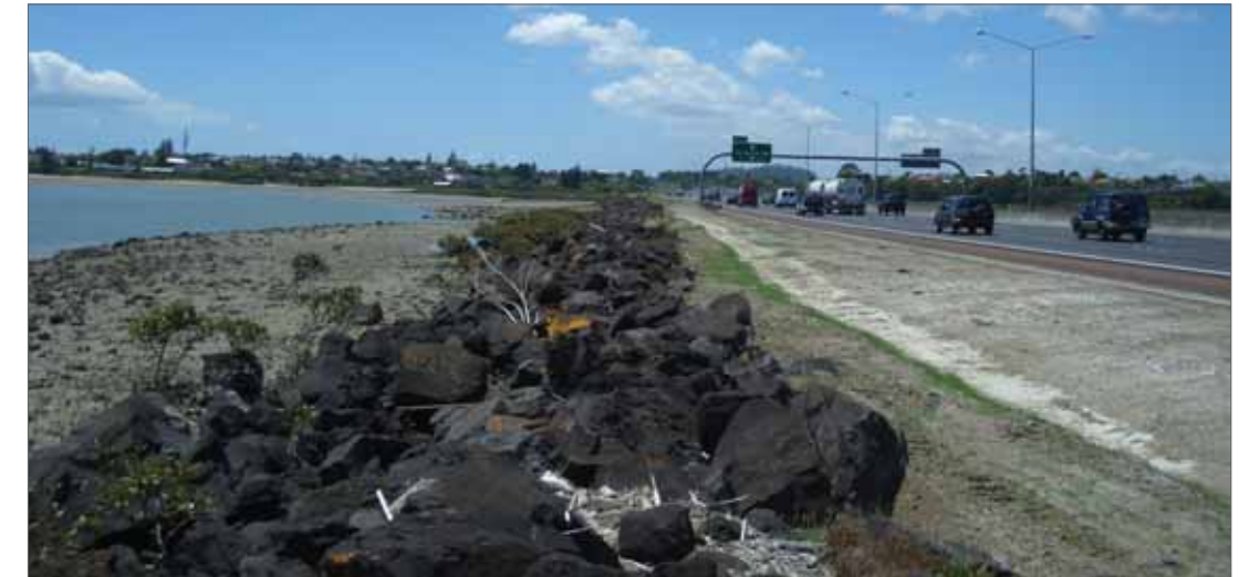
Figure C-4.7: Photo 4-3 Existing view eastwards approaching Rosebank bridge
