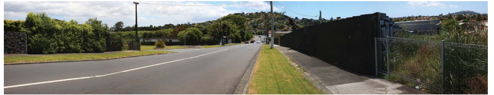
Figure C-9.7: Photo 9-7 View down Richardson Road towards Stoddard Road shops (proposed Richardson Road bridge location)
