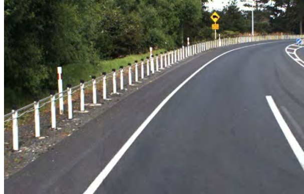
Photo 16: Wire rope barriers used on road side
