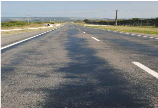
Photo 1: Flushed or slippery section located within wheel track. Source: Yvonne Forrest (MOTO).
