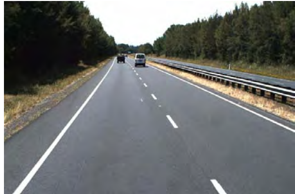
Photo 14: W-beam or steel barriers
