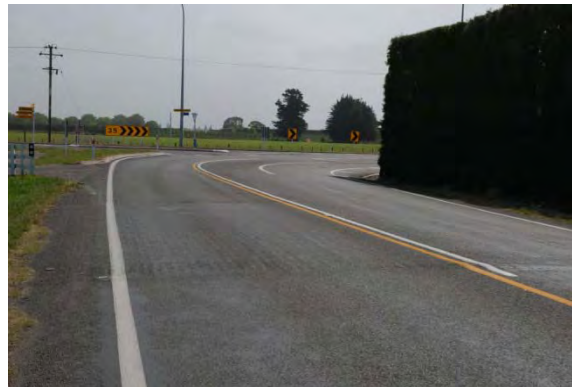
Photo 4: Seal change located in brake zone. Source: Yvonne Forrest (MOTO)
