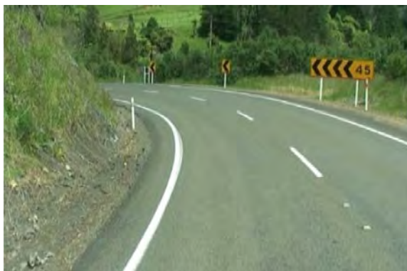
Photo 9: Delineation treatment, SH 2 Waioeka Gorge. Source: Opus Consultants
