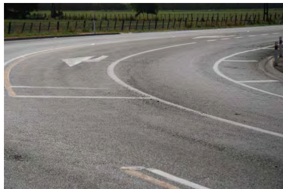
Photo 3: Gravel migration located on a curve. Source: Yvonne Forrest (MOTO)
