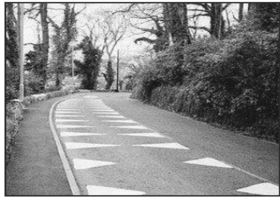
Photo 24: Perceptual countermeasures to slow speeds on approach to an urban area ( Dragon's teeth) Charlton and Bass, (2006)
