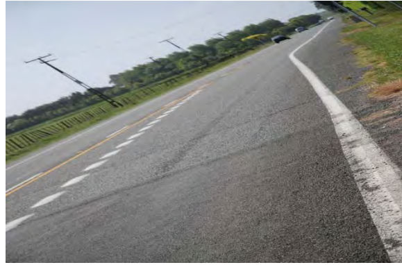
Photo 6: Removal of obsolete road markings. Source: Yvonne Forrest (MOTO)
