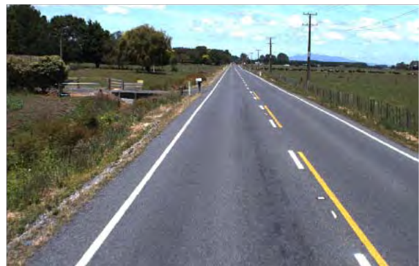
Photo 12: Steep slopes and open drains located within clear zones
