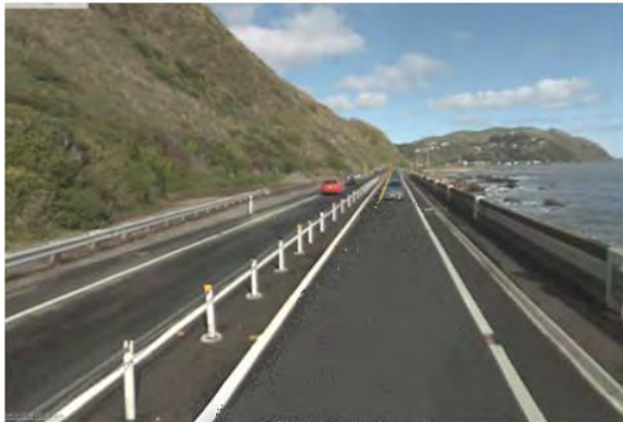
Photo 15: Wire rope barriers used in centre
