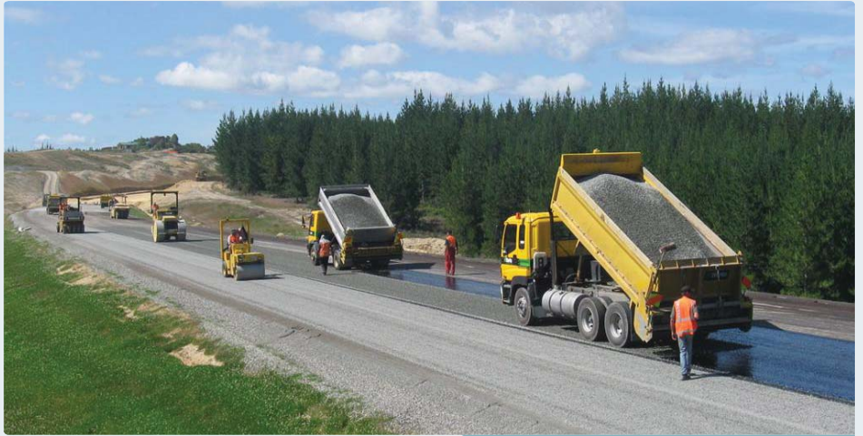
Laying the 'first coat seal' earlier this year
