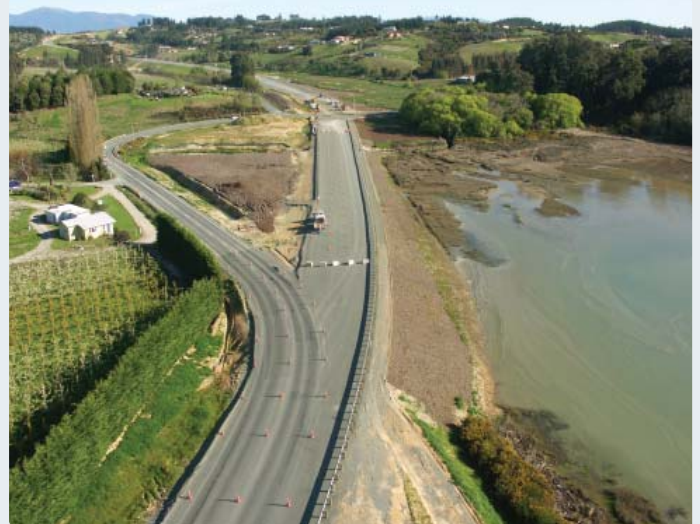
The new alignment nearing completion 2010
