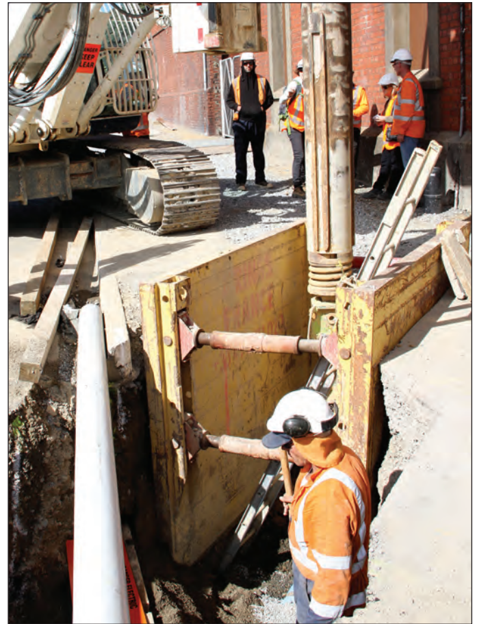
2013: A careful operation is needed to move the pipes out of the way. At left, the vacuum cleaner sucks up slushy soil with a hose. At right, the ground at the sides is held in place by retaining walls so workers can put in a new water pipe.
