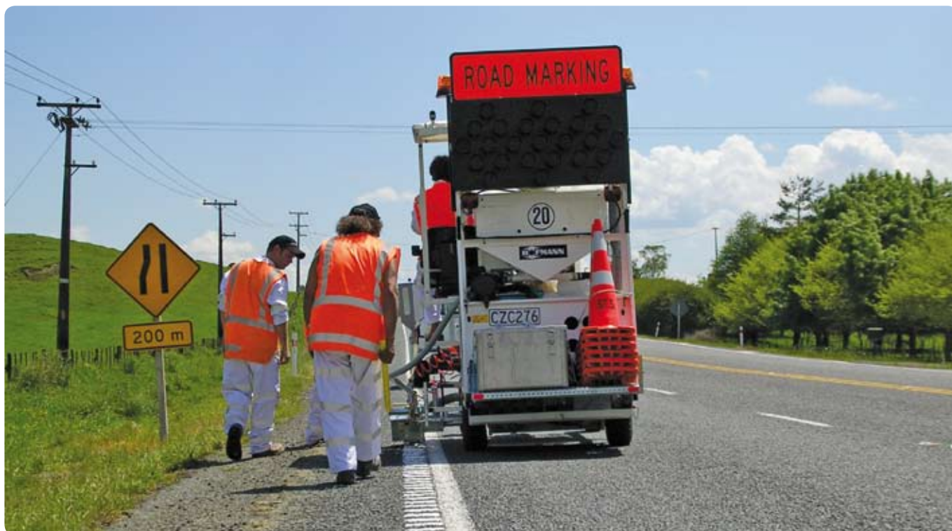
The NZTA will install around 750 kms of rumble strips before June 2009
