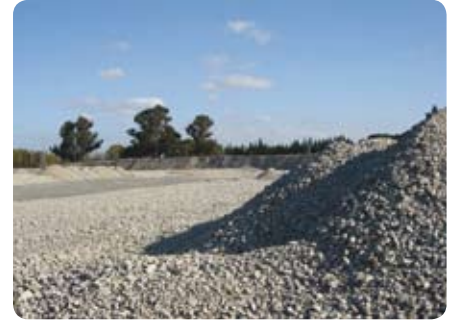
Stockpiled recycled crushed concrete for the Christchurch Southern Motorway.
