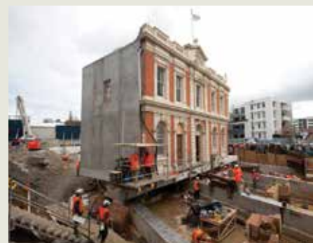
PREPARING THE ROB ROY HOTEL FOR ITS HISTORIC MOVE.
