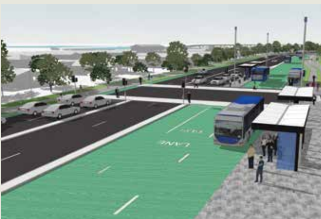
PAKURANGA ROAD BUSWAY - PART OF THE PROPOSED BUSWAY FROM PANMURE TO PAKURANGA. BUS STOPS ARE AT INTERSECTIONS TO IMPROVE SAFETY FOR PEDESTRIANS.
