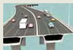
7 COMPLETED NEW NEWMARKET VIADUCT
