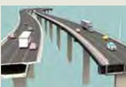
4 NEW 4 LANES SOUTHBOUND IN USE
