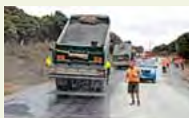
⌘ STATE HIGHWAY 1 – WAITIKI LANDING TO CAPE REINGA PROJECT.
