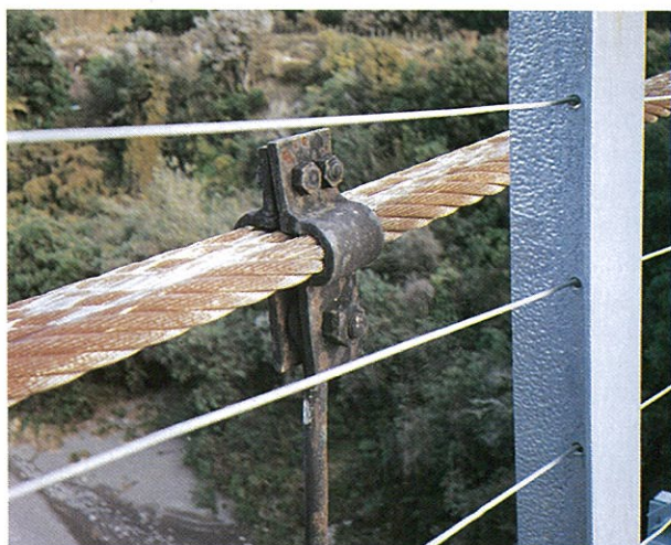
Figure 4.12: Pitted steel posts refurbished by galvanizing.
