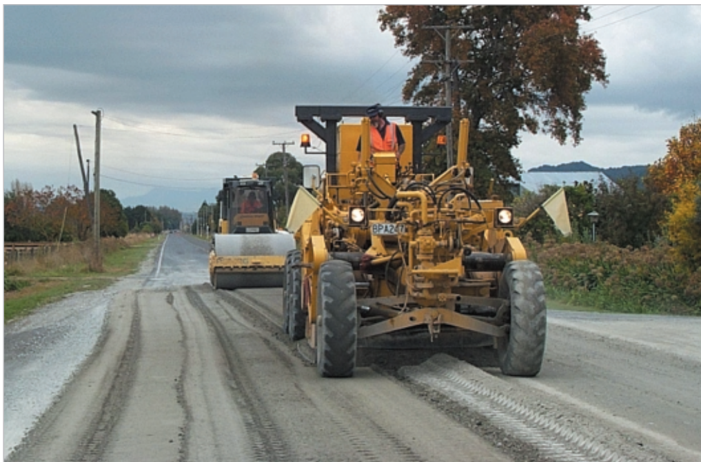
Figure 12-9 Recycling a multiple chipseal that has developed layer instability.
