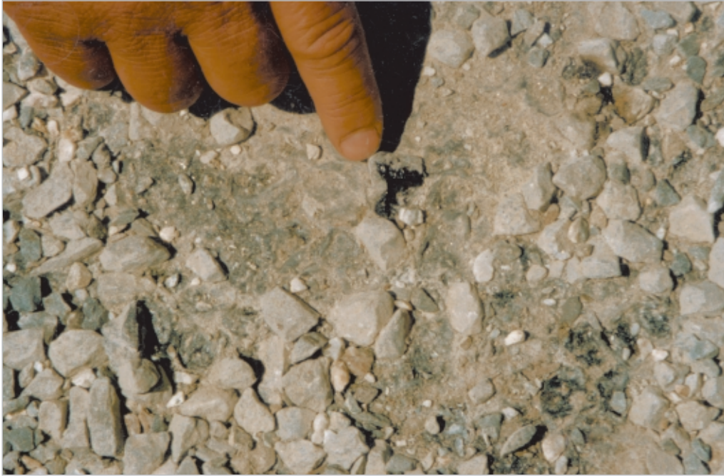
Figure 12-4 Chip loss caused by dirty chip in the seal.
