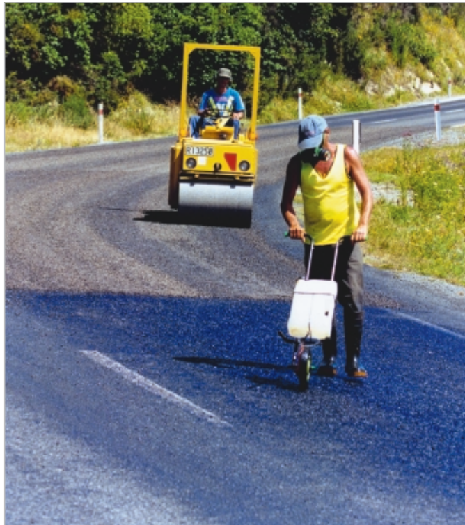
Figure 12-6 Solvent (e.g. kerosene) being applied before it is covered with chip.
