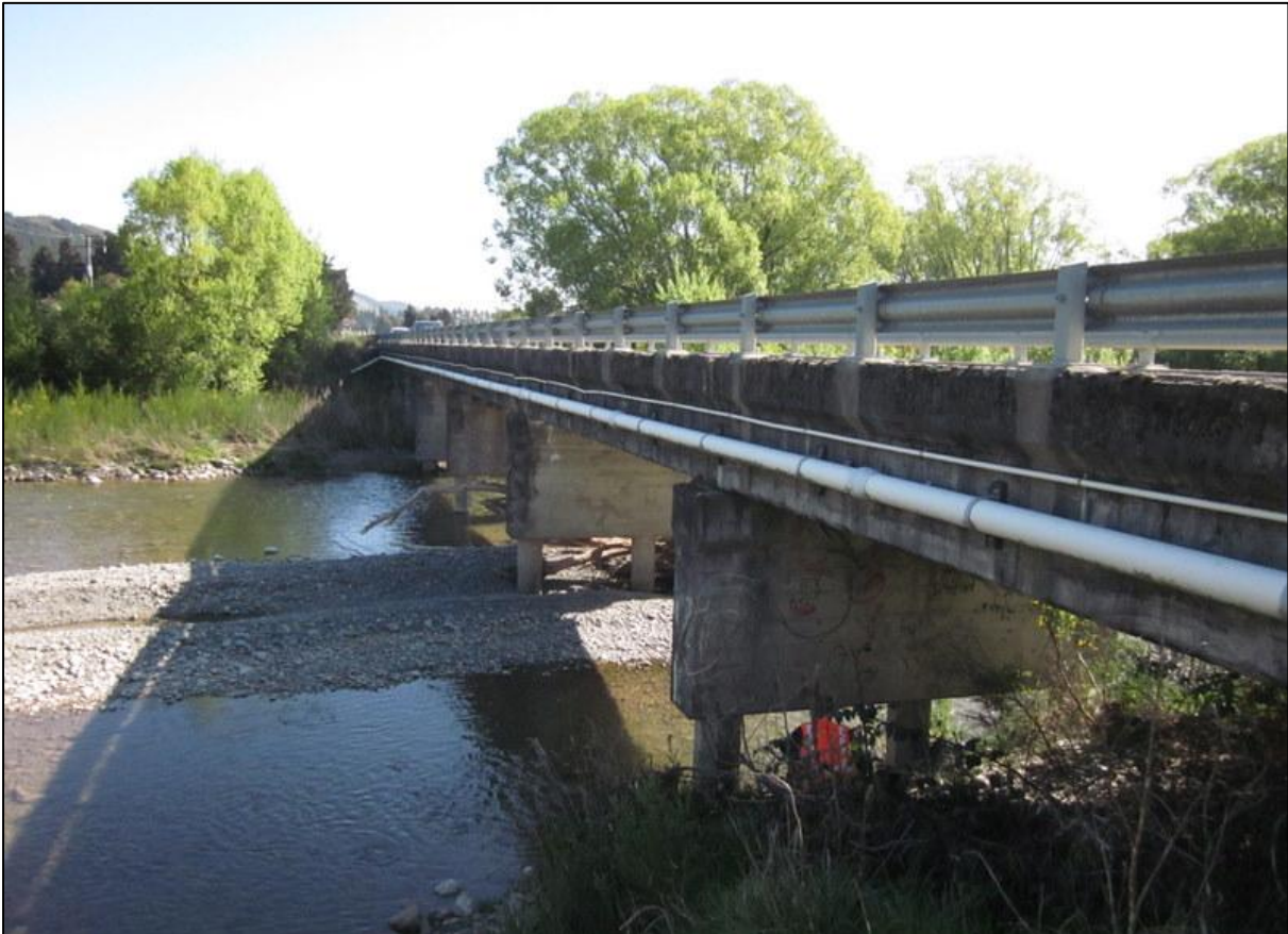
SH77 Selwyn River Bridge, looking south-west.
