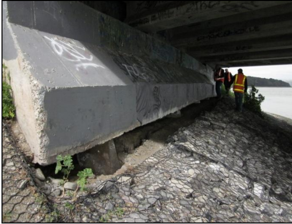
Figure BS1 Settlement at east abutment.
