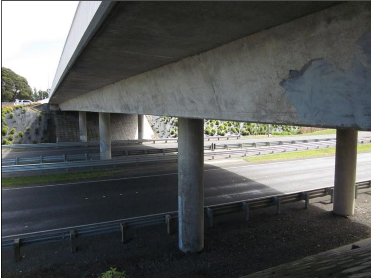
Ohoka Road Underpass, looking west.
