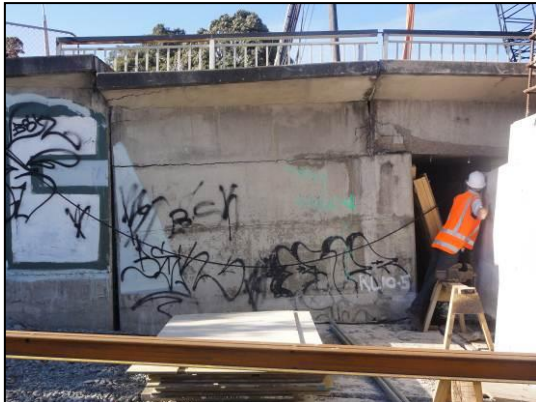
Figure 10. CCC Ferrymead Bridge. Lateral spreading damage to abutment wall and piers in the 22 February 2011 Christchurch earthquake.
