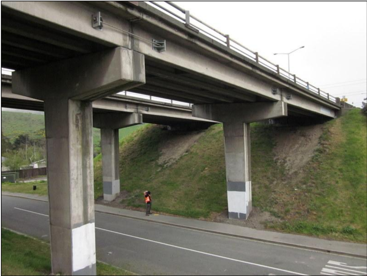
SH74 Horotane Valley Overpasses Nos 1 and 2, looking west.
