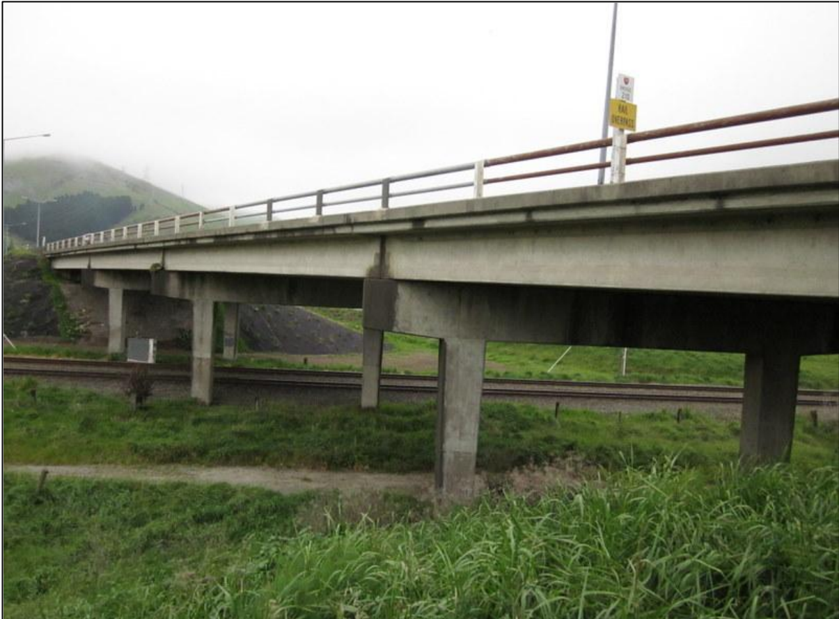
SH74 Railway Overbridge, looking south.
