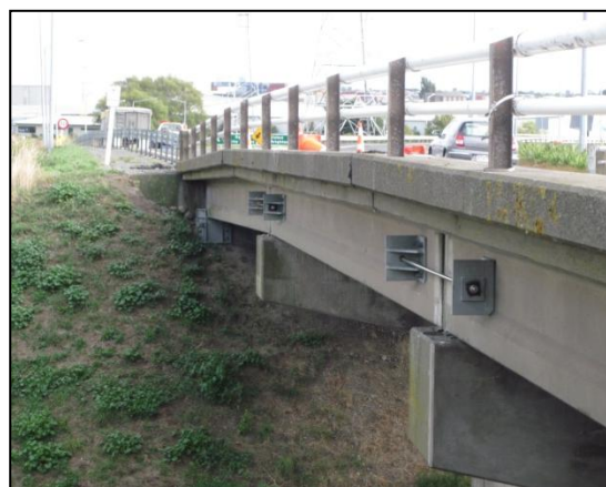
Figure HO2 Settlement of abutment at city end.
