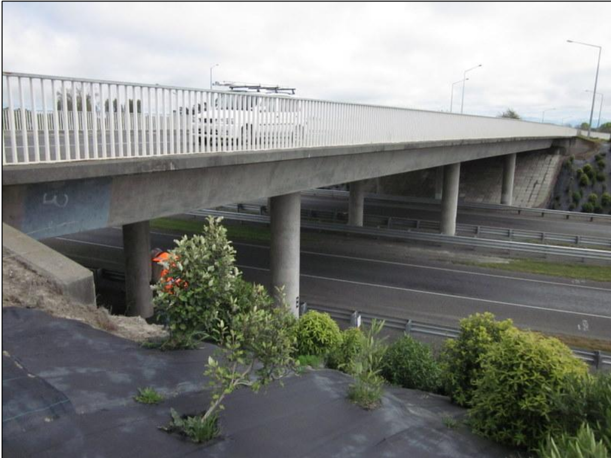
SH71 Cam Road Underpass, looking east towards Kaiapoi.
