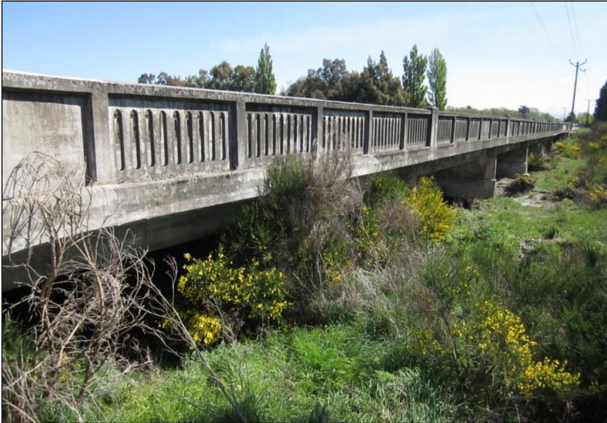
SH77 Hawkins River Bridge, looking west.
