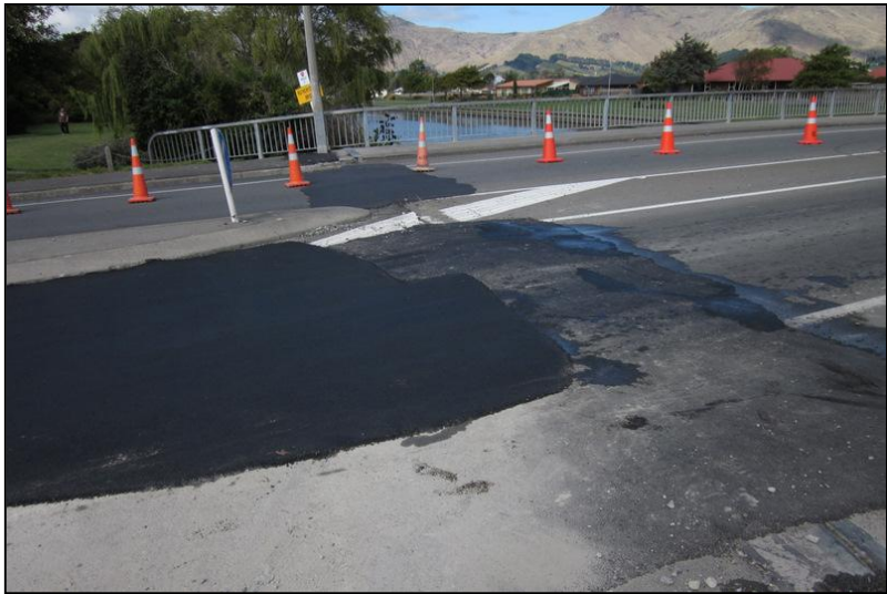
Figure R1 Closed deck joint at north abutment.
