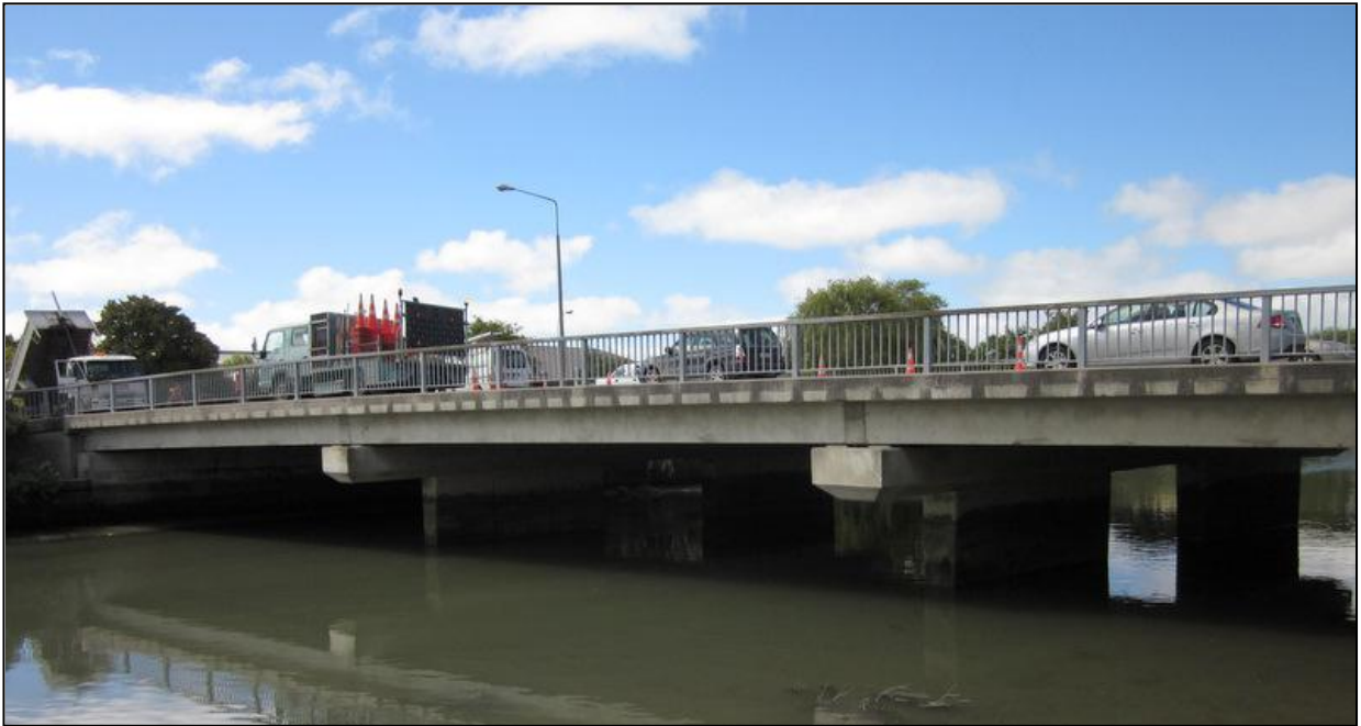
SH74A Rutherford Street Bridge, looking north-east.
