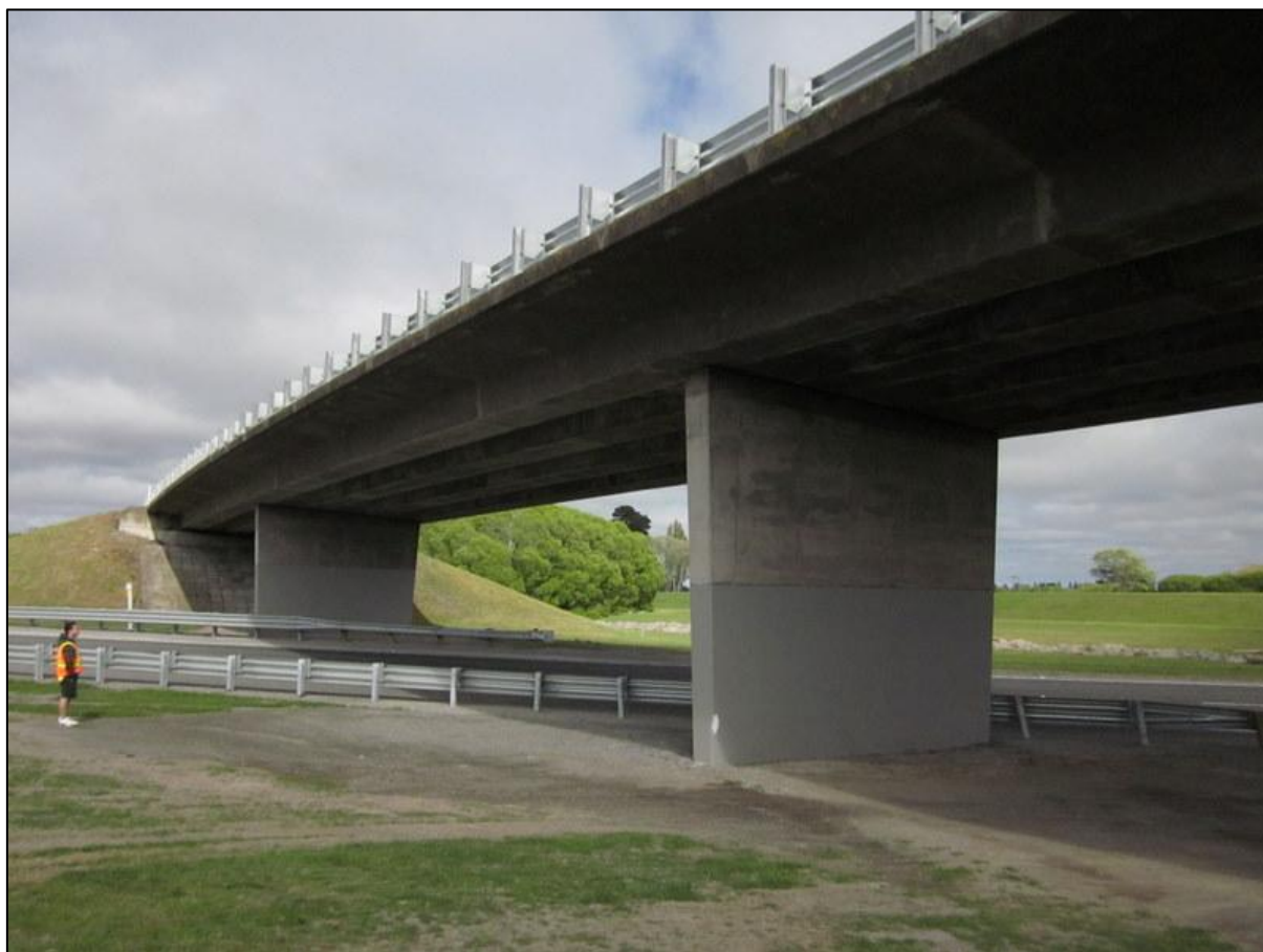
SH1 Chaney's Road Overpass, looking south-west towards Christchurch.
