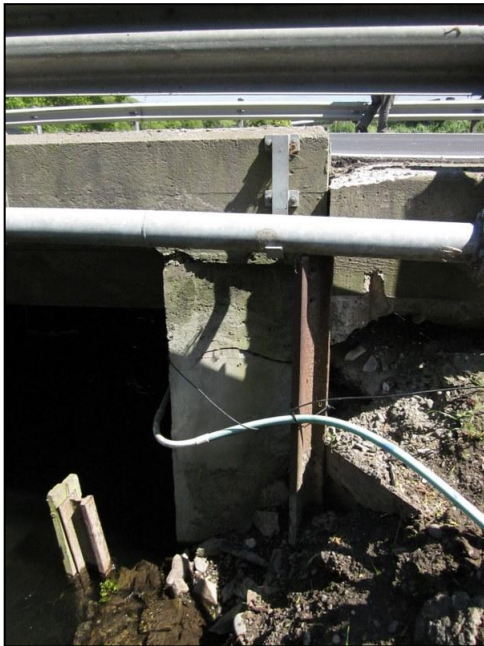
Figure H1 North-east corner.
