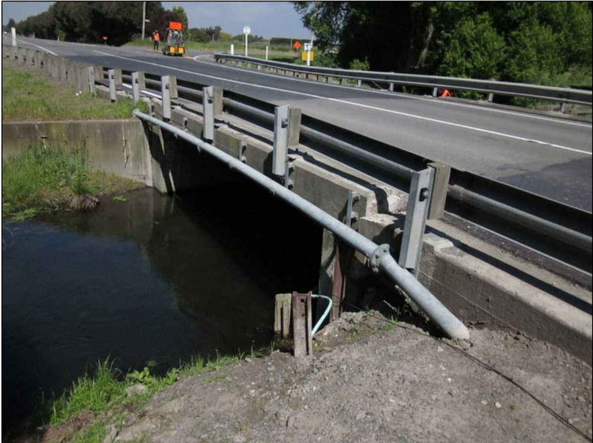
SH75 Halswell River Bridge (Landsdown), looking south.
