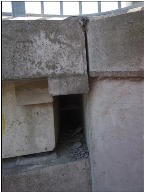
Figure R1 Closed deck joint at north abutment.
