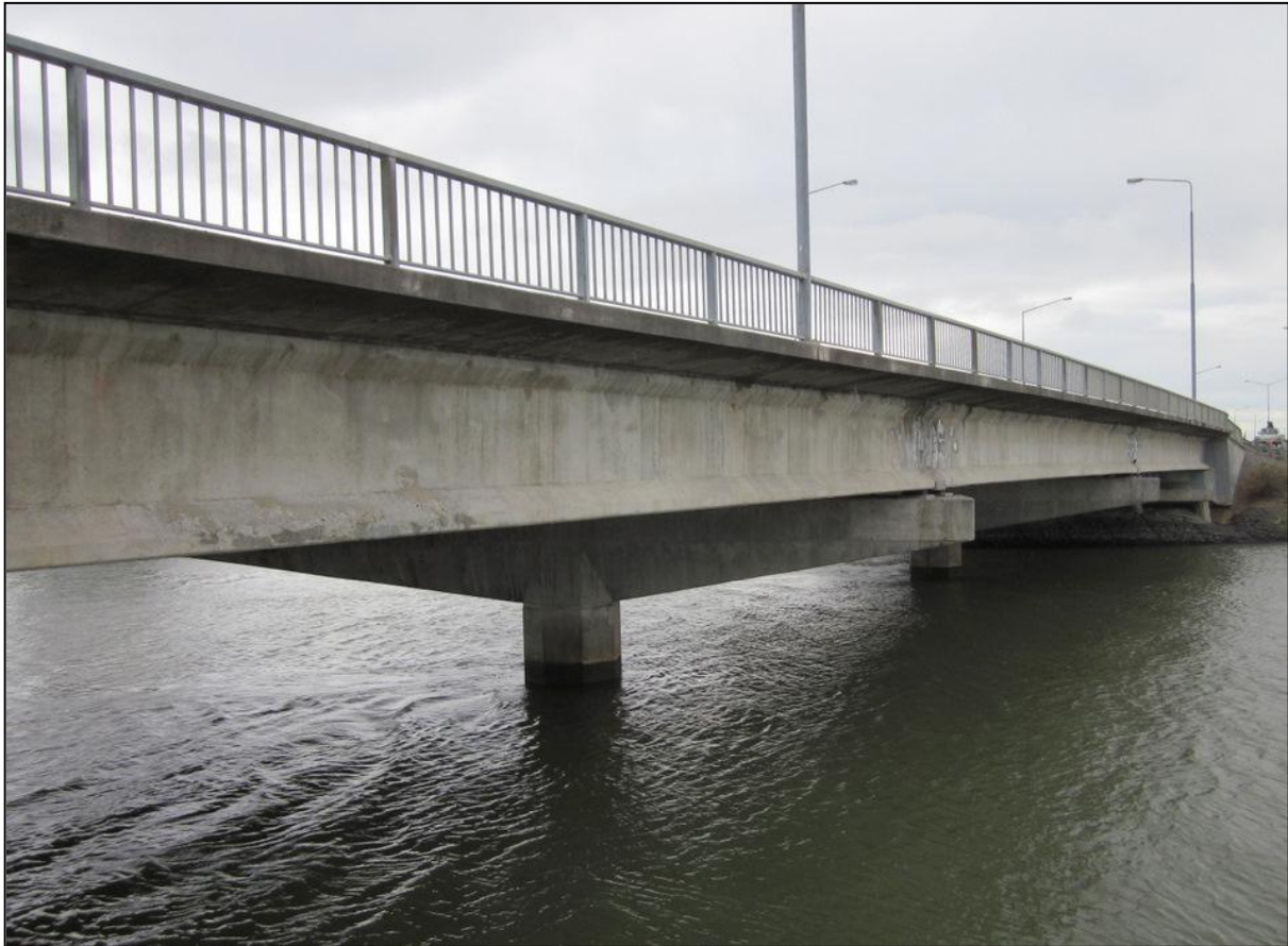
Bridge Street Bridge, looking west.
