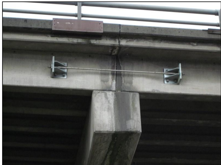
Figure HO6 Linkage bolt at pier.
