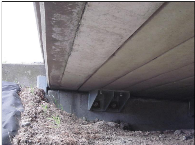
Figure PH3 Abutment shear keys.
