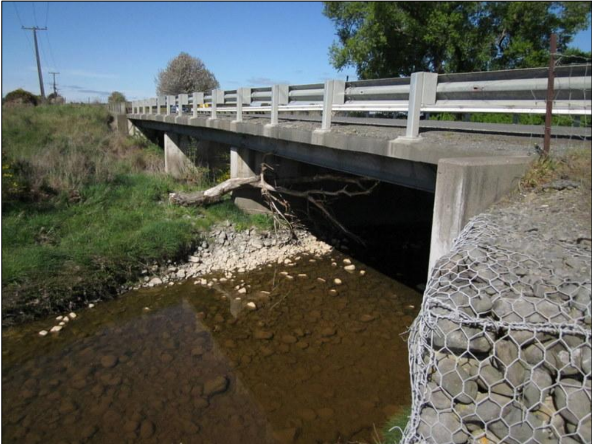
SH77 Waianiwaniwa River Bridge, looking east.
