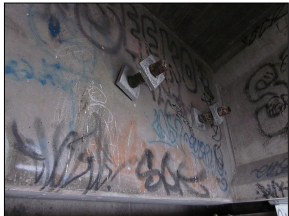
Figure BS4 Bearing displacement at east abutment.
