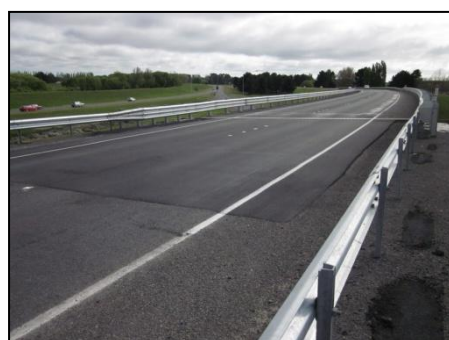
Figure C5 Repaired pavement at north approach.
