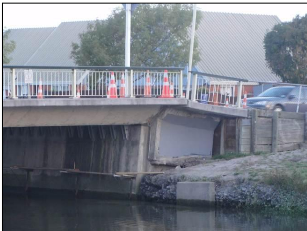
Figure 10. CCC Ferrymead Bridge. Lateral spreading damage to abutment wall and piers in the 22 February 2011 Christchurch earthquake.
