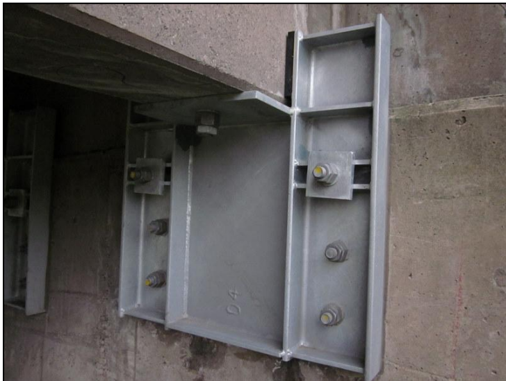
Figure HO5 Shear key at abutment.
