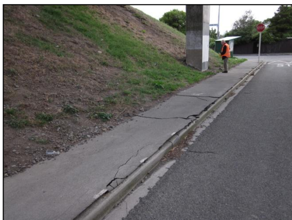
Figure HO2 Settlement of abutment at city end.
