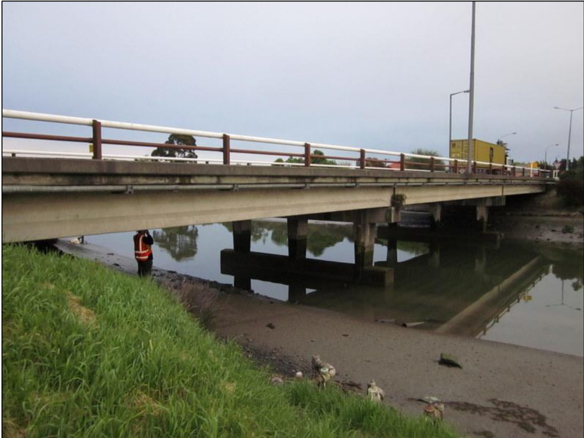
SH74 Heathcote River Bridge, looking north-west.
