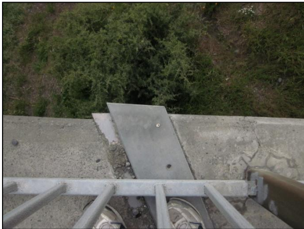
Figure BS1 Settlement at east abutment.
