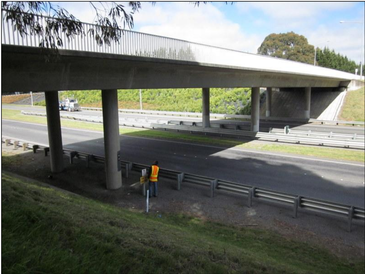
Tram Road Underpass, looking west.
