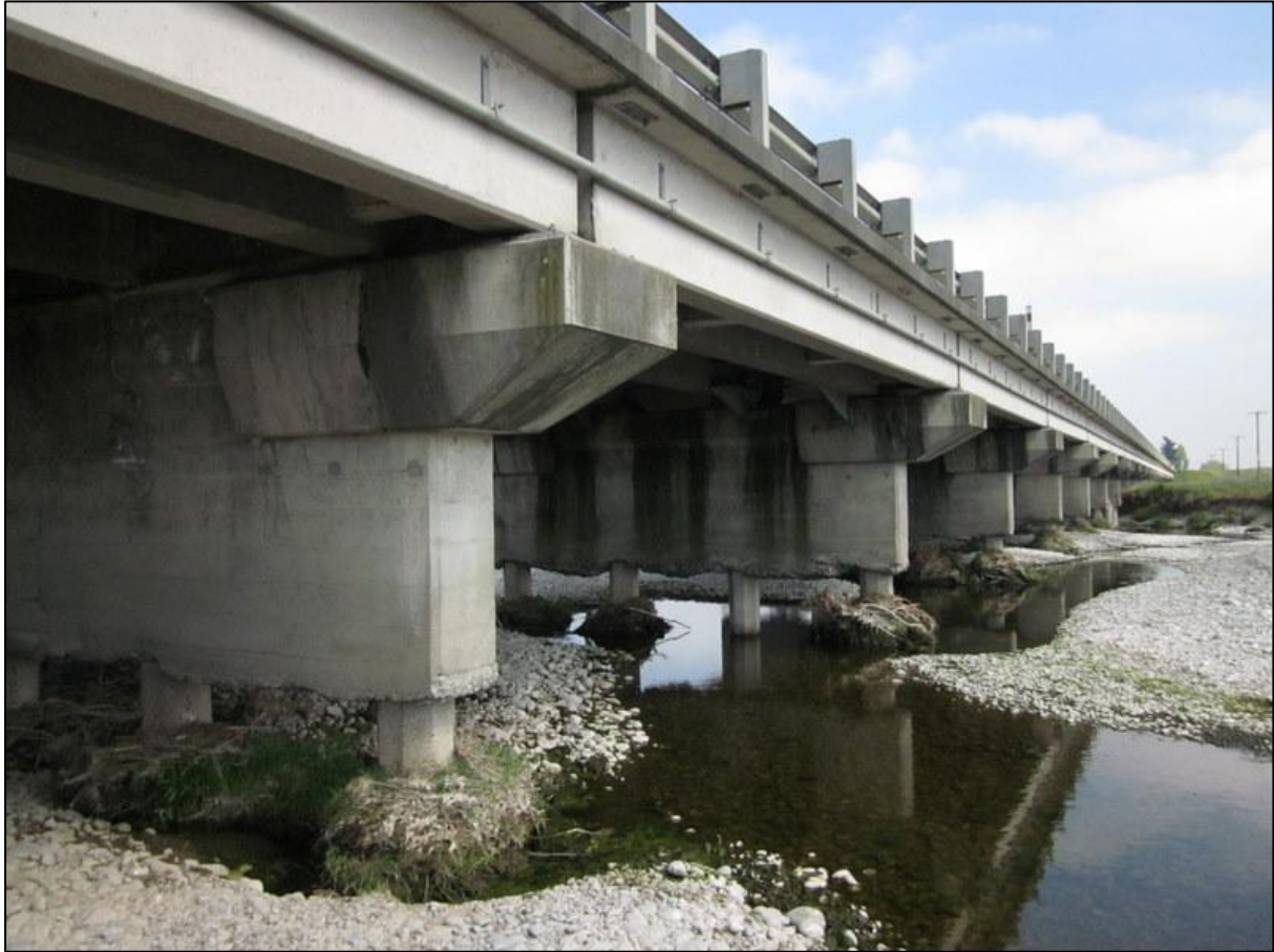
SH1 1 Selwyn River Bridge, looking north. (Northern spans of thirty five.)
