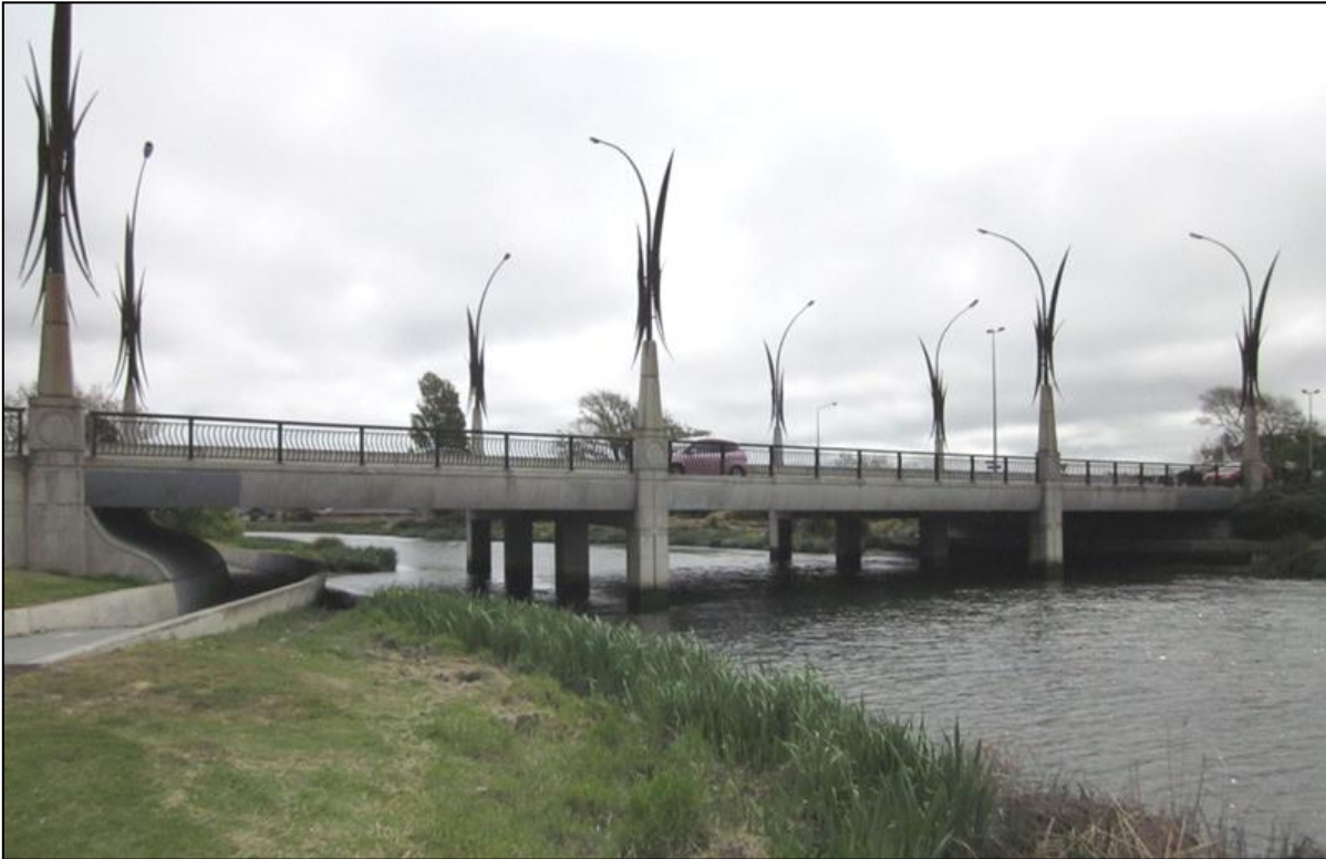
SH74 Anzac Drive Bridge, looking north-west – 14 October 2010.
