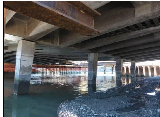
Figure 10. CCC Ferrymead Bridge. Lateral spreading damage to abutment wall and piers in the 22 February 2011 Christchurch earthquake.
