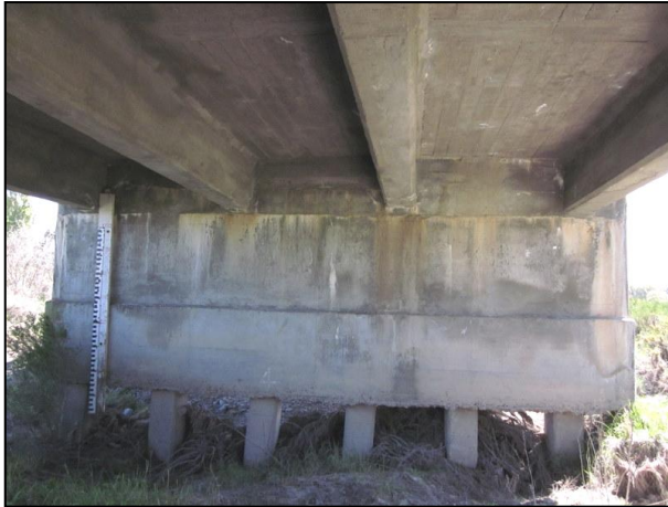
Figure HA1 Pier and piles.
