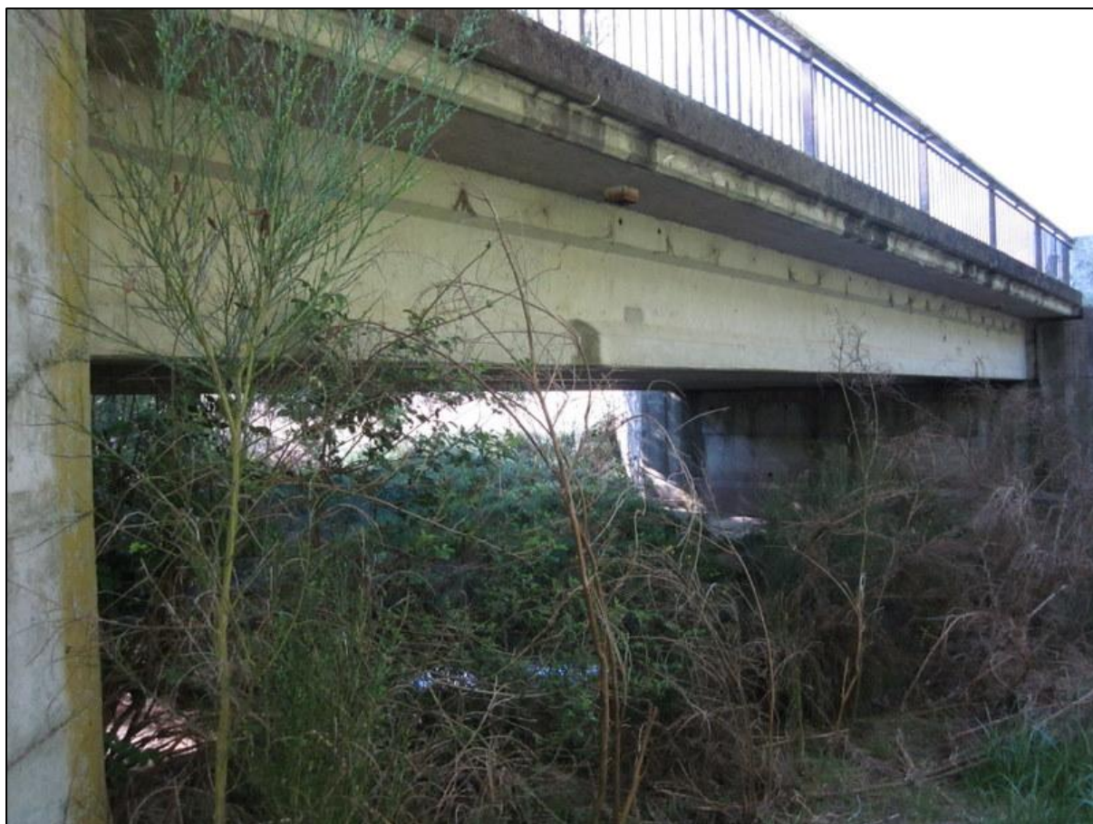
SH77 Wairiri Stream Bridge, looking north.
