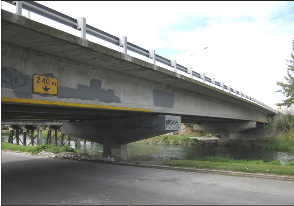
SH73 Heathcote River Bridge (Opawa) looking south-east.
