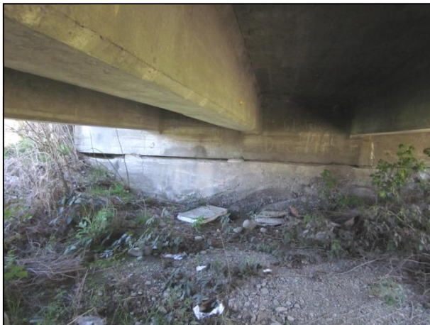
Figure HA3 Infill concrete below west abutment.
