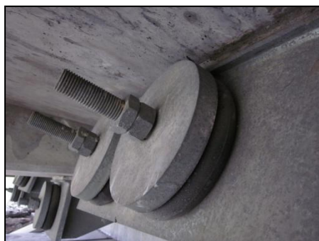
Figure C1 Linkage bars at north abutment.
