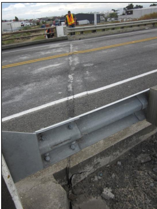
Figure RO1 Deck joint at north abutment.
