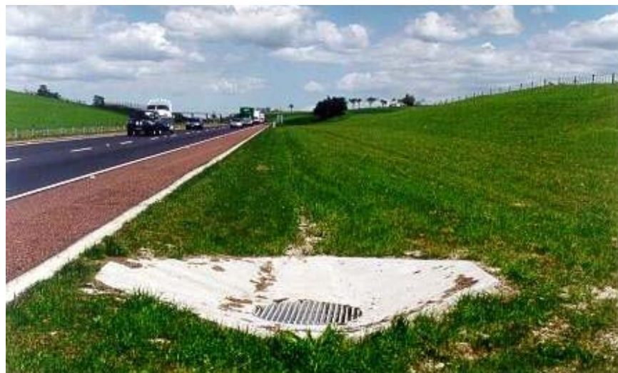
A vegetated swale on this site, Auckland South Western Motorway, State Highway 20 is consistent with a number of Transit's expectations for highway landscaping
