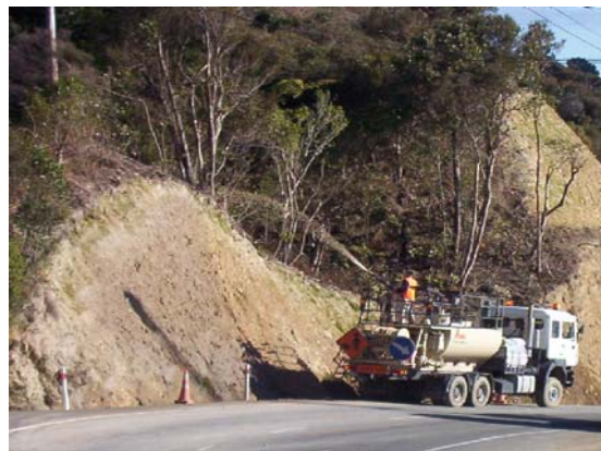
Hydroseeding at Kaitoke, State Highway 2
