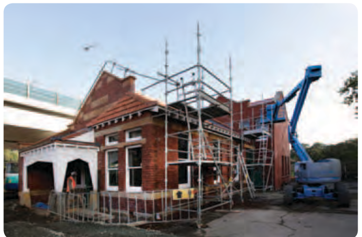
Campbell Free Kindergarten nearing restoration
