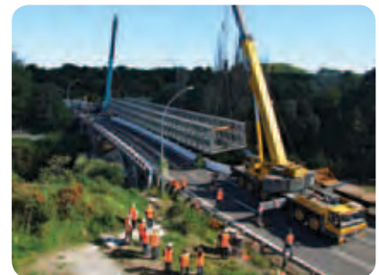
The temporary Bailey bridge is removed at Narrows Bridge
