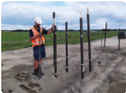
Monitoring of trial embankments for the Tauranga Eastern Link Project
