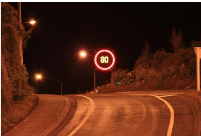
Figure 7.2 Variable speed limit sign indicating 80km/h speed limit applicable at the time
