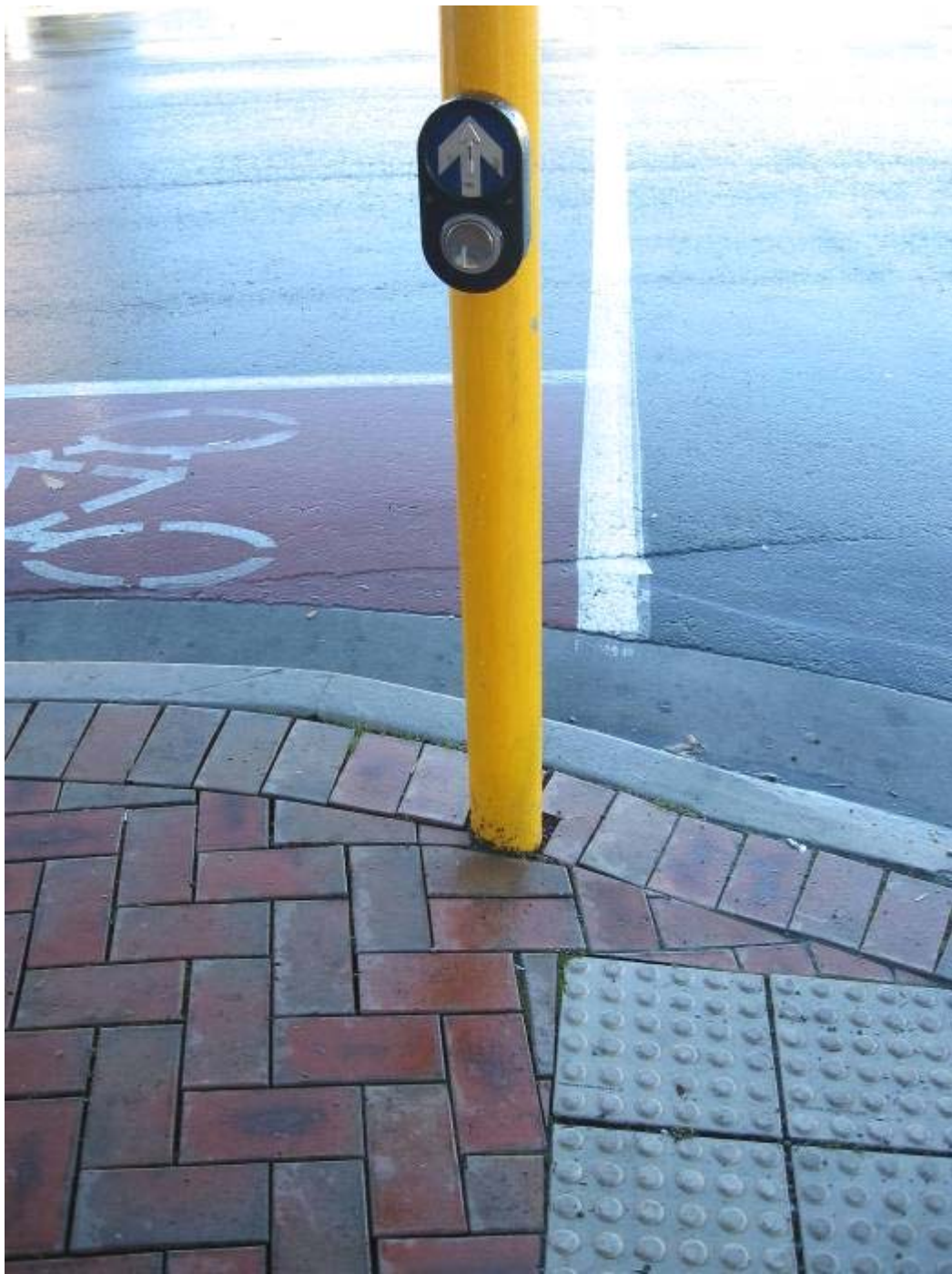
Photo 16. This installation is an example of best practice with the warning TGS and pedestrian call box both aligned with the crossing direction. The gap between the TGS and signal pole is so small that a person cannot inadvertently enter the road without receiving tactile warning.
