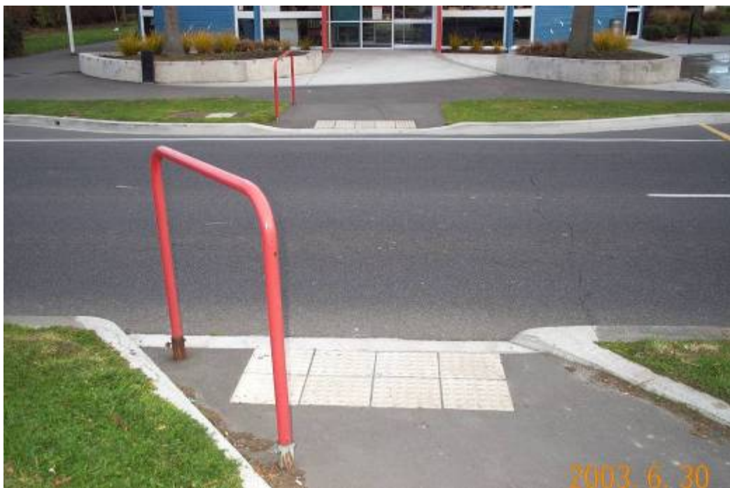
Photo 12: The warning indicators are aligned with the road crossing direction. (Note again: not quite full width)
