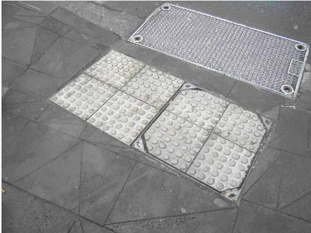
Photo 20: An example of how warning TSGI can be integrated into the design of utility service cover.
