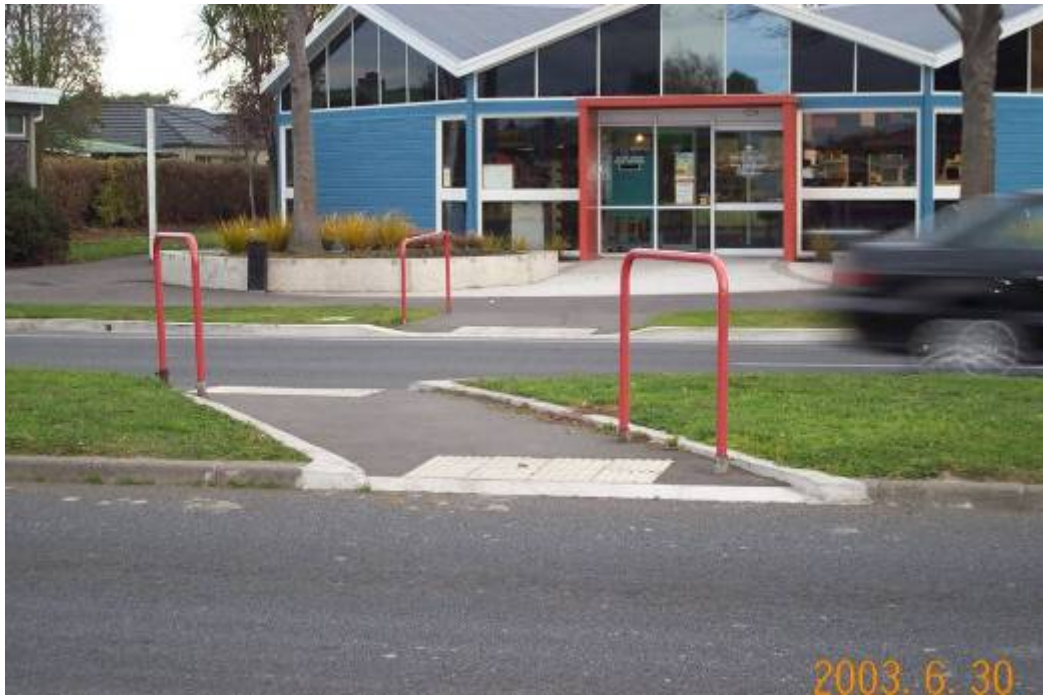
Photo 11: On deep medians, two sets of warning indicators are installed. (Note: again not quite full width.)
