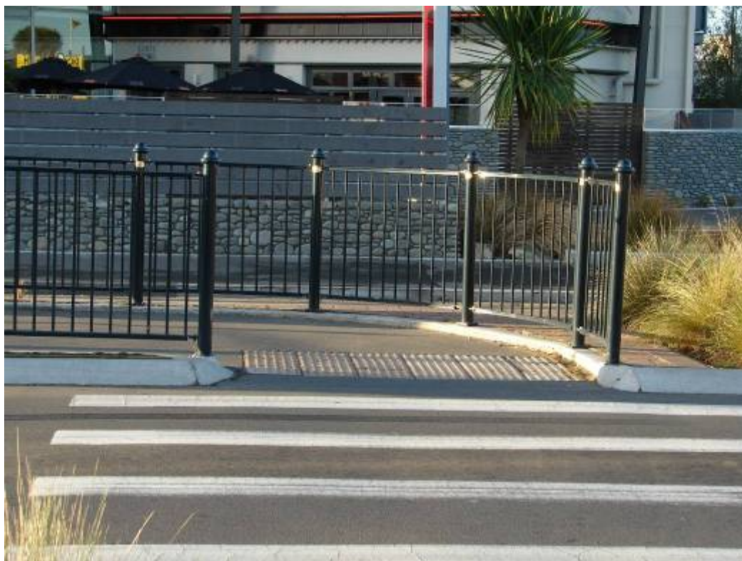
Photo 13: Example of a staggered median crossing with marked pedestrian crossing over the traffic lanes.
