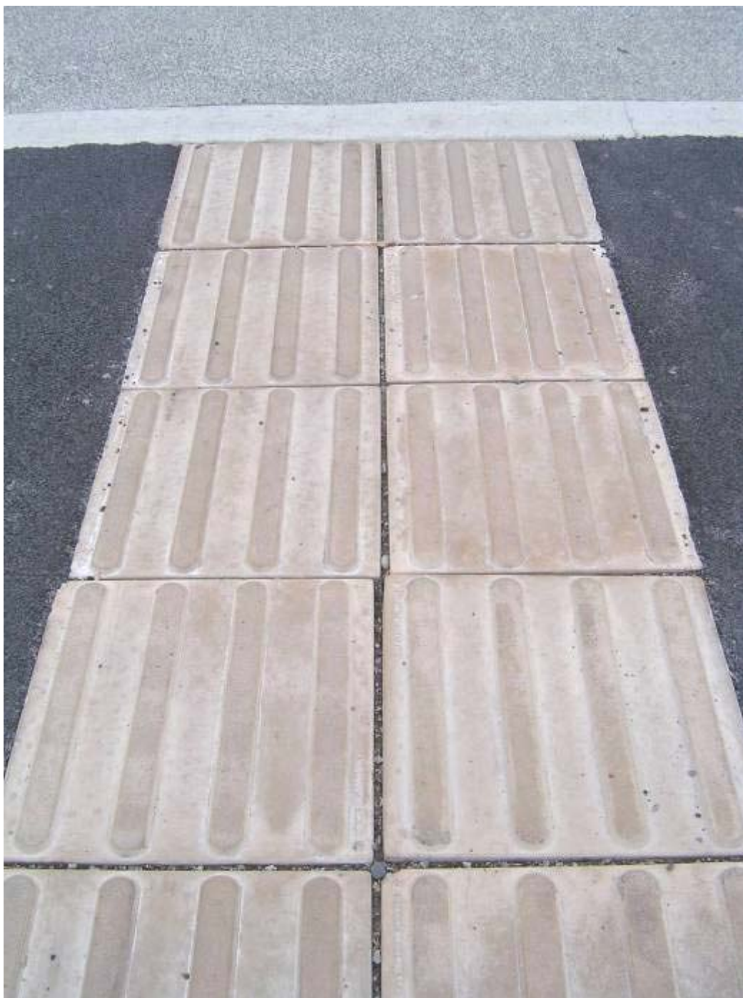
Photo 6: View of directional indicators.
