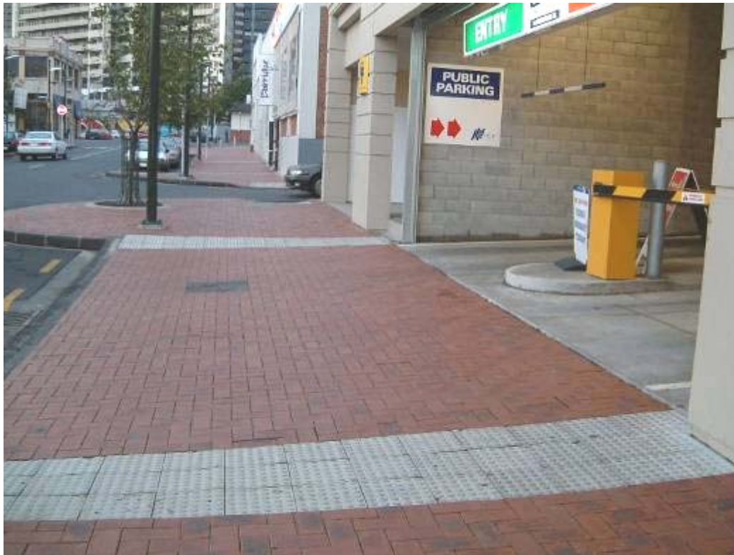
Photo 24: Warning indicators extend across the full width of the footpath outside a car park building.
