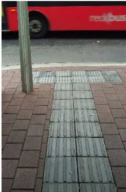
Photo 23: Directional indicators lead to warning indicators at a bus stop.
