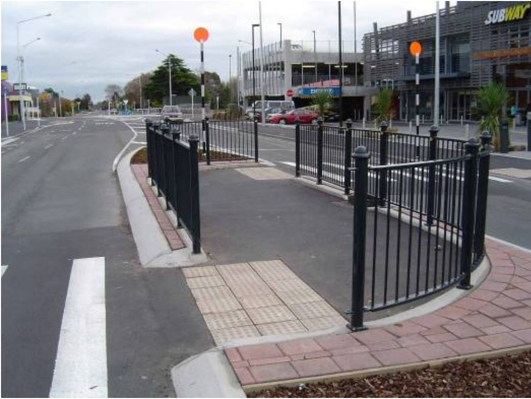
Photo 14: The kerb and fencing provides tactile cues within the staggered median to assist vision-impaired pedestrians.
