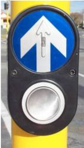
Photo 19: Pedestrian push-button assembly.
