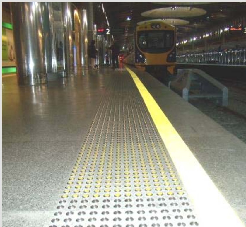
Photo 7: The warning indicators at this railway station are 600mm deep and set 600mm back from the platform edge. A better photo is to be sourced because the contrast is marginal and not uniform.
