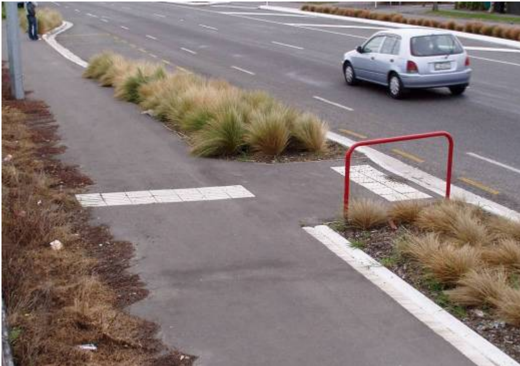
Photo 8: The directional indicators shown in this installation cover the full width of the path while other features, including the planting and a handrail provide tactile cues to the road crossing point.
