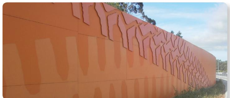
A section of barrier with visible joints and artwork inspired by vehicle tyre-tracks.
