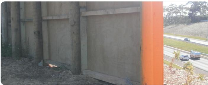
Construction issues are evident on this barrier: the rear of the barrier is unpanelled and unpainted, and gaps show between the barrier and the ground.
