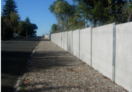
Directly before planting, topsoil and mulch implemented
