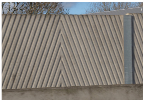
Patterned section of the wall
