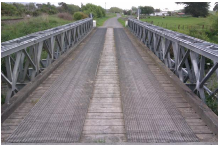
Bridge A – Otauru Road
