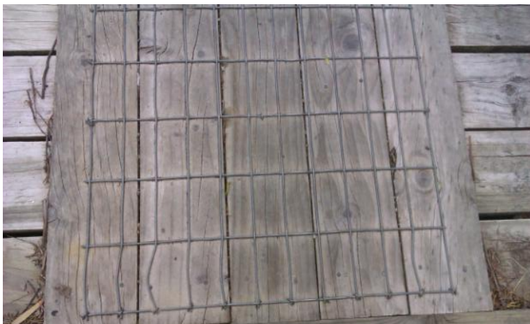
Bridge B - Metal mesh on running surface
