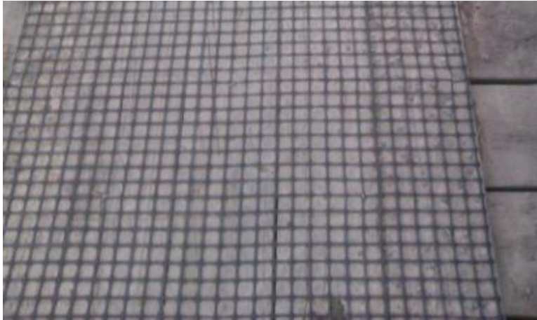
Bridge A - Plastic mesh on running surface
