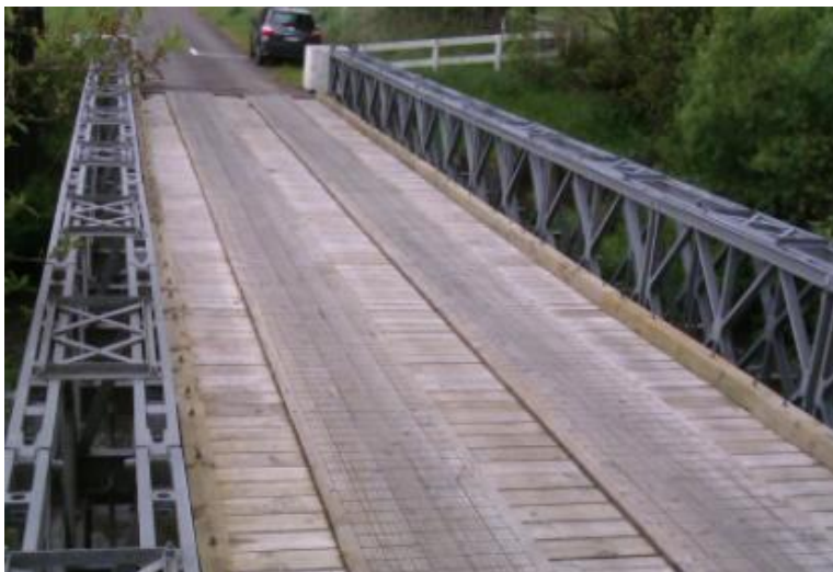
Bridge B - Hennessey Road
