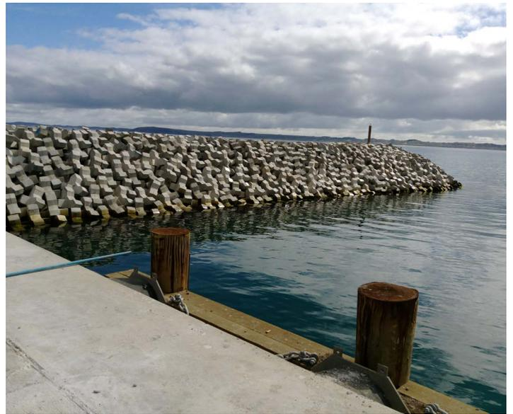
The construction of the wharf structure and breakwater armour required approximately 100,000m<sup>3</sup> of rock aggregate and sand materials.
