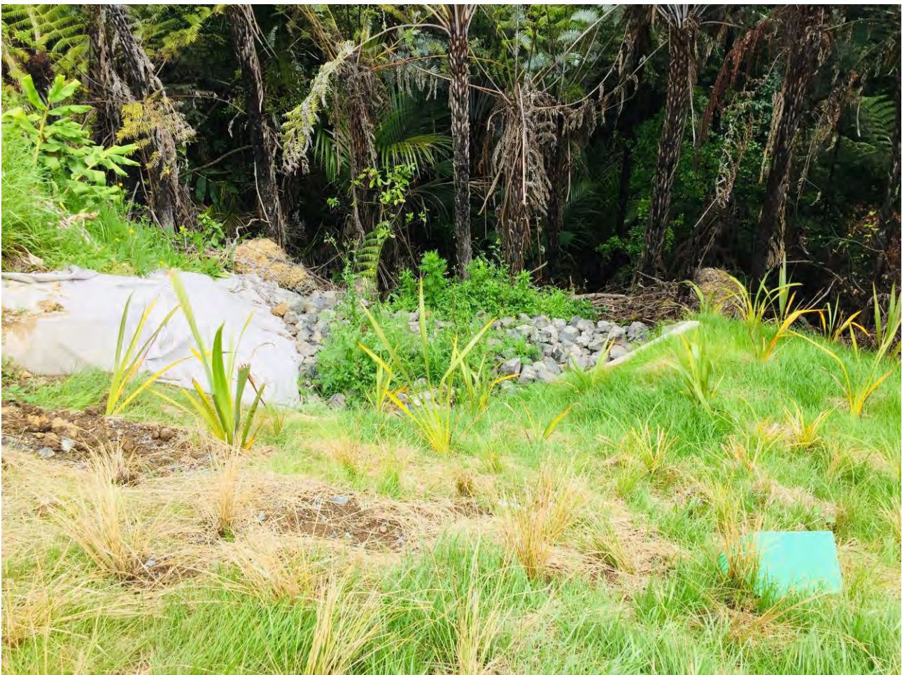
Figure 6: Existing cross drainage discharge area with riprap and non-recoverable slopes with grown vegetables
