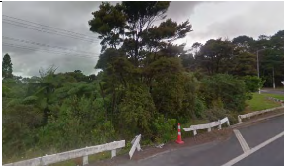
Figure 19: Existing broken sight rails along the Dairy Flat Highway after the T-intersection Silverdale leg.
