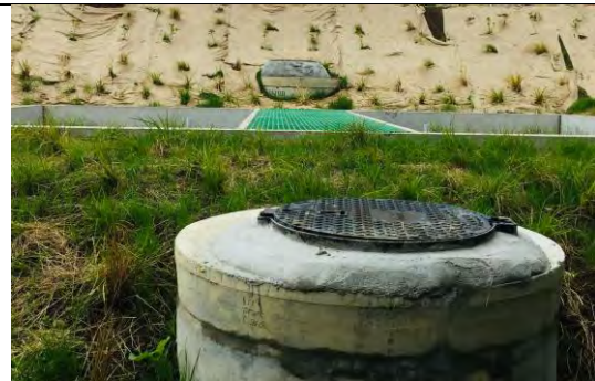
Figure 13: Existing stormwater system and fill slope.
