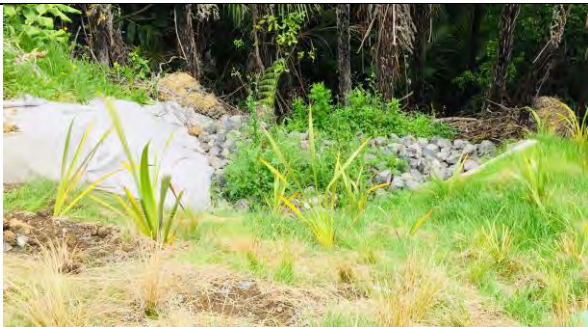
Figure 12: Stormwater discharge area with riprap and grown vegetations.
