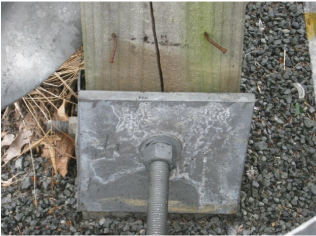
Bearing plate slipped around
