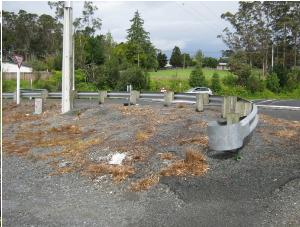
Curved Rail and Trailing End Terminal
