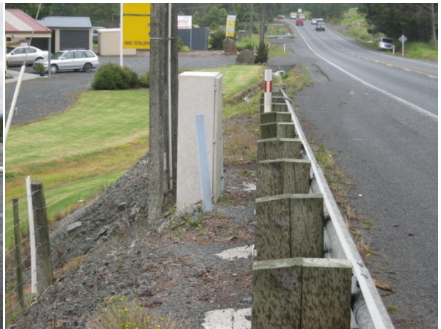
North end steep batter unprotected
