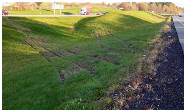
**Figure 2: A used clear-zone on the roadside**
