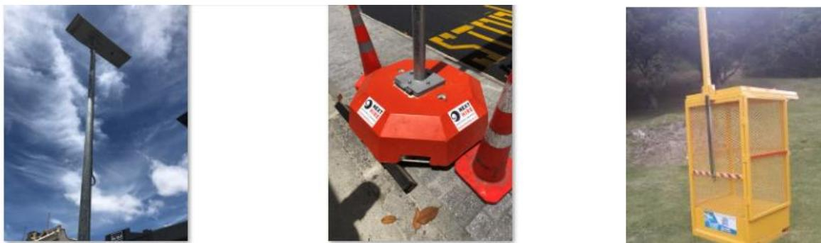
**Figure 35: temporary lights (L to R) - overhead pole, concrete base mount (Auckland), cage mount (Tauranga)**
