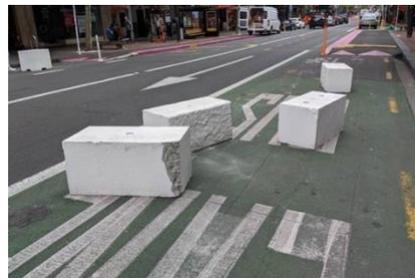
**Figure 4: concrete separators dislodged, Auckland**
