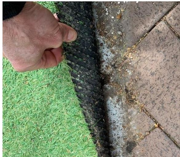
**Figure 34: not all edges are traversed by pedestrians - glue may be sufficient, Nelson**
