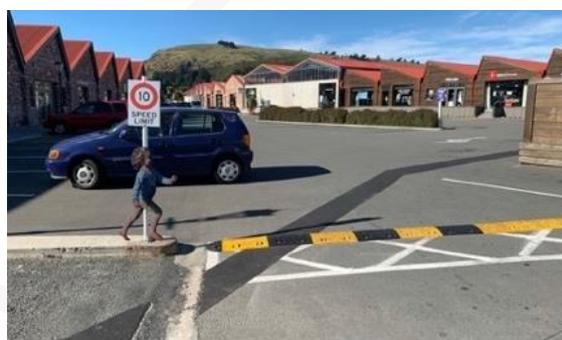
**Figure 24: rubber speed hump and child crossing figure; speed limit sign non-compliant (J. Lieswyn)**
