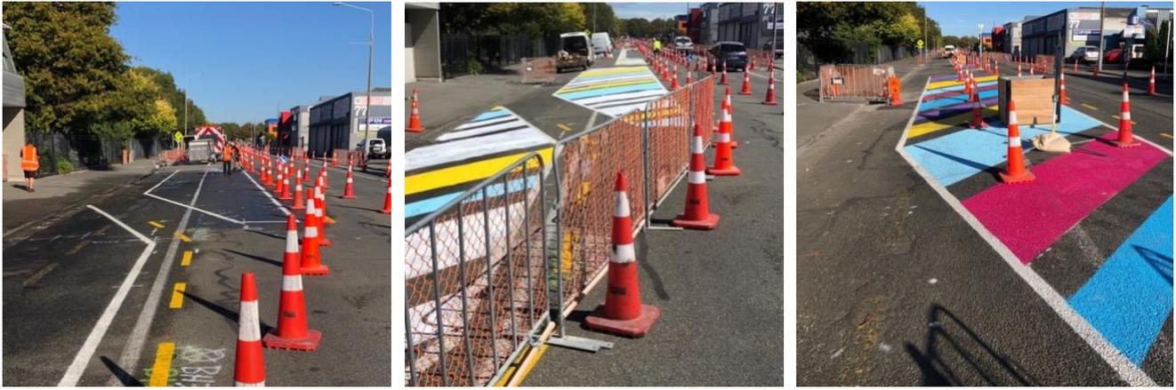
**Figure 30: clean the surface, apply white primer, finish coat. Standard paint with grit mixed in is used as the surface is not going to be trafficked, Christchurch (C. Piper)**
