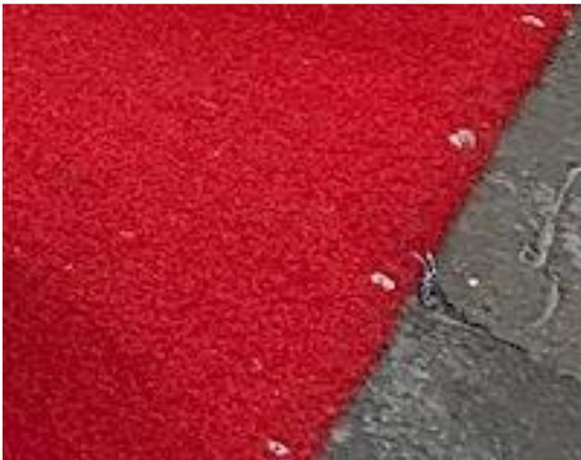
**Figure 33: glue and screws used on asphalt provides for heavy skateboard and pedestrian traffic, Nelson**
