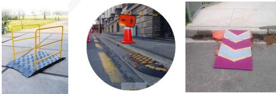
**Figure 22: temporary ramps may be made of rubber, wood or asphalt (latter not pictured); must be slip resistant**
