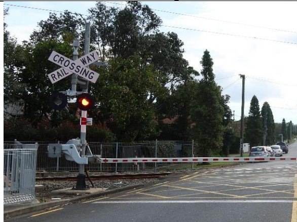
View of signalling when crossing is activated on the correct side of the road
