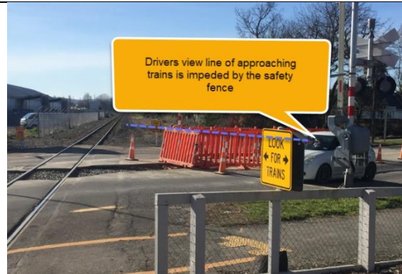
Example of driver view lines where fencing is used in proximity to the rail corridor
