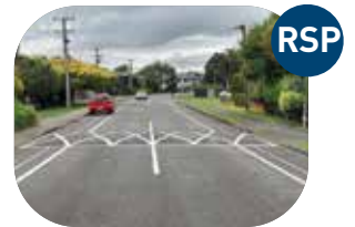
Construct Hump/ platform
