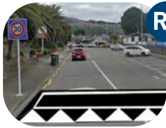
Raised Threshold Treatment
