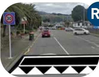
Raised Threshold Treatment
