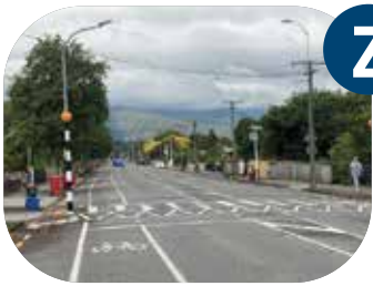
Reconstruct existing Zebra Crossing on Raised Safety Platform
