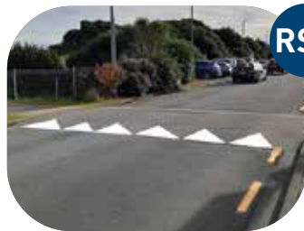
Construct Raised Safety Platform
