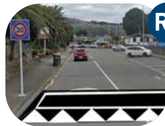
Raised Threshold Treatment
