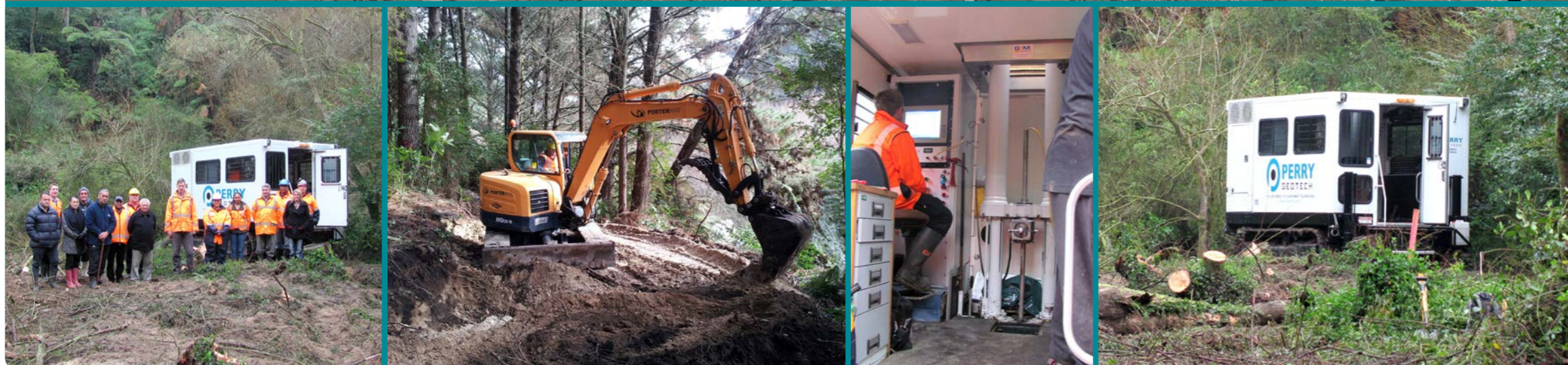
Karapiro Stream Gully blessing prior to geotechnical investigations
