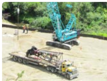
Progress in Karapiro Gully
