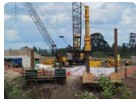
Piling under way at southern abutment of Karapiro Viaduct
