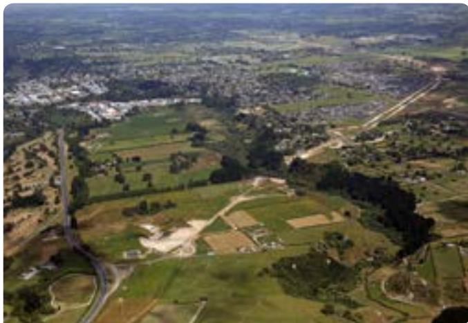
View of the Expressway alignment from the south
