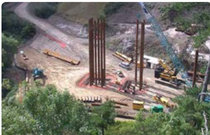
Viaduct piling work in Karapiro Gully
