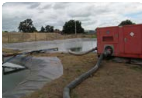
Temporary water pond at Peake Road
