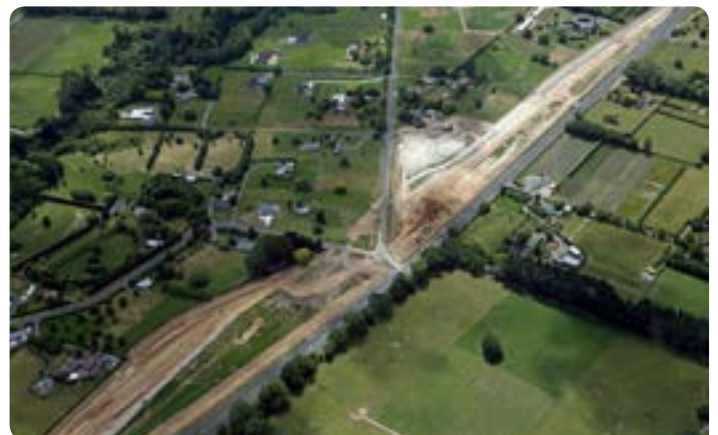
Progress at the north end of site, Pickering Road
