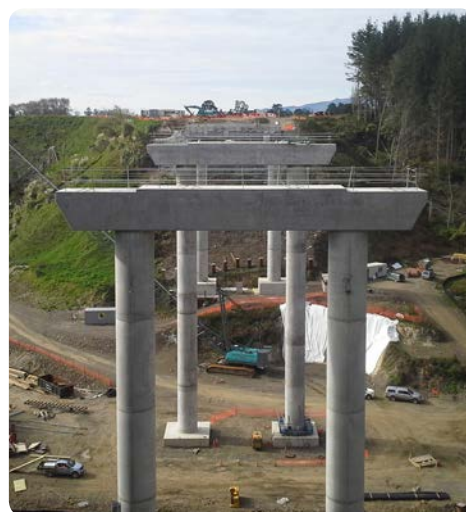
Karapiro Gully viaduct progress.
