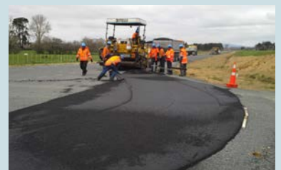
Paver laying asphaltic concrete
