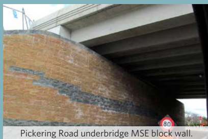
Pickering Road underbridge MSE block wall.
