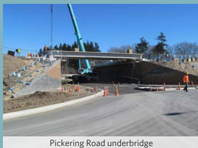
Pickering Road underbridge
