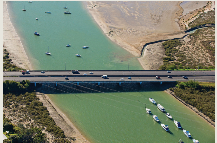
Whau River Bridge
