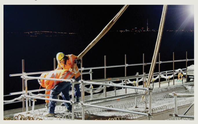
Above: Team members Nick and 'Stretch' unhook a beam after placement, photographed by Safety, Health and Environment Advisor, Brigitte. Two Super T beams can been seen in the centre of the photo below, now firmly encased in concrete.
