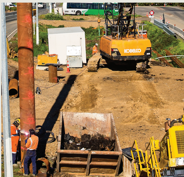
Patiki piling crew - specialist welders joining the pile casings (bottom left) on site for the deep piles.
