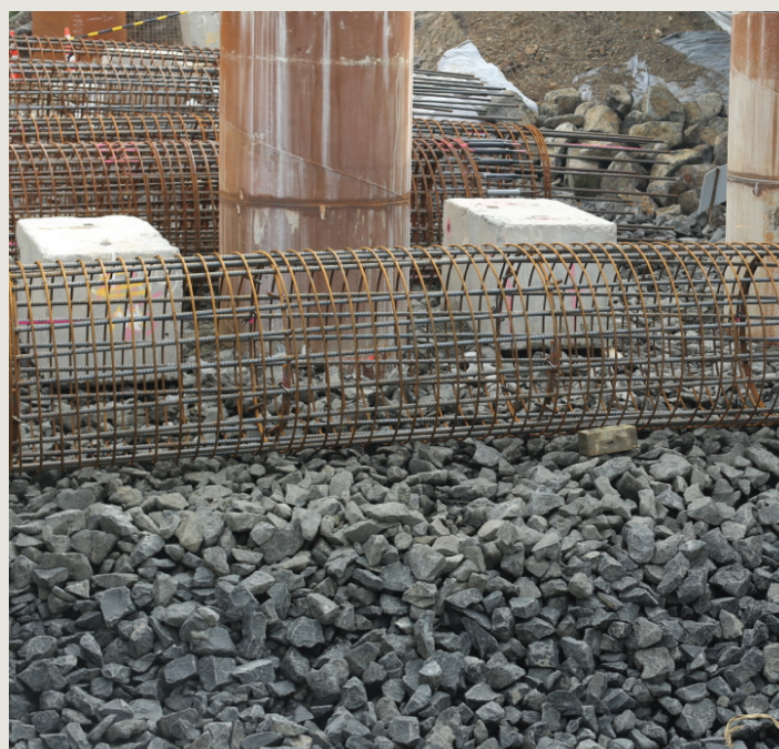
Reinforcing steel cages which are lowered into the pile casings.
